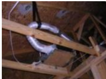
Poor installation (U bend)
