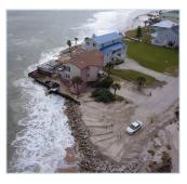
Along the north shoreline of St. Augustine Inlet, the Porpoise Point area has experienced significant erosion, exposing the end of Porpoise Point Drive to hydrodynamic impacts from storms and waves. Despite multiple sand placement events by St. Lucie County on the east end of Porpoise Point Drive, the sand has washed away and further exposed the road
