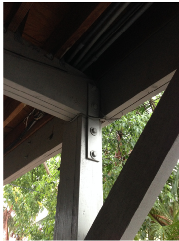
(Pic.3) Typical Perimeter Roof Support
