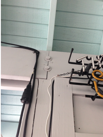
(Pic. 10) Upstairs bar wood beam (Inadequate connection)
