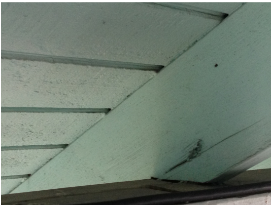
(Pic.12) Upstairs bar roof rafters (No visible roof uplift connections)
