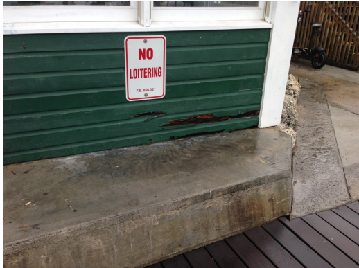
(Pic. 1) Exterior cladding (Deterioration from moisture)
