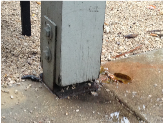
(Pic.6) Wood column post at covered walkway (Gap at base)
