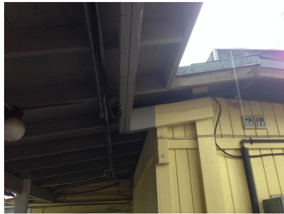
(Pic.7) Inadequate beam support at walkway canopy structure
