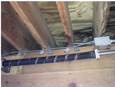
(Pic.4) Typical Roof Framing (2x12 spaced at 12" o.c.)
