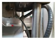
**Location:** Kitchen **System:** Electrical **Condition:** Conduit Not Properly Connected **Explanation:** The conduit as installed is not properly connected to a panel or junction box.
