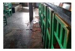
**Location:** Interior Bar **System:** Interior **Condition:** Trip hazard in floor surface **Explanation:** The floor surface has an abrupt change in height where different floor finishes abut. This condition has a variation that is sufficiently great as to present a potential trip hazard.
