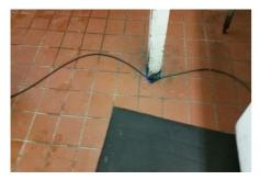
**Location:** Kitchen **System:** Electrical **Condition:** Unsafe Wiring Installation **Explanation:** Distribution wiring is installed in an unsafe manner or location. **Impact Consequences:** Electrical wiring installed in an unsafe manner or location may pose a risk of fire or shock hazard. Consult a licensed electrician for proper installation of the observed wiring.
