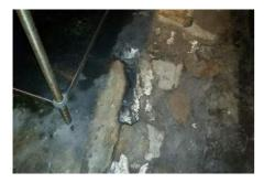
**Location:** Interior Bar **System:** Interior **Condition:** Trip hazard in floor surface **Explanation:** The floor surface has an abrupt change in height where different floor finishes abut. This condition has a variation that is sufficiently great as to present a potential trip hazard.
