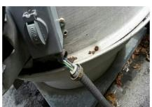
**Location:** Roof **System:** Electrical **Condition:** Conduit Not Properly Connected **Explanation:** The conduit as installed is not properly connected to a panel or junction box
