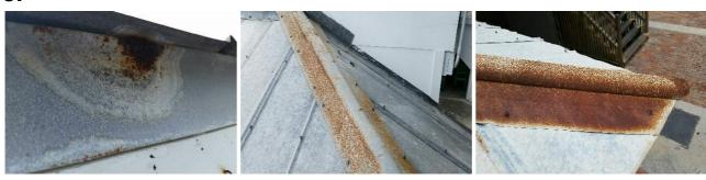
Location: Roof System: Roof Condition: Metal roofing is rusted Explanation: The metal roof covering is observed to have areas of rust. Impact Consequences: Areas of rust are an indication that the metal roofing is near or past its useful life expectancy and replacement should be considered as the most effective form of action. Rust often leads to perforation and leaks; surface repairs typically provide only short-term protection.
