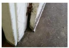
**Location:** Kitchen **System:** Exterior **Condition:** Exterior door is deteriorated **Explanation:** The overall condition of an exterior door is observed to be deteriorated such that its operability and performance characteristics are impaired. Exterior door operation and performance considerations include: ability to restrict forced entry; ability to open and close with relative ease; ability to securely close and latch; ability to restrict entry of air water and pests.
