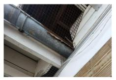
**Location:** Lower Dining Deck **System:** Roof **Condition:** Gutter is deteriorated **Explanation:** A gutter is observed to be in a deteriorated condition. Repairs are required to restore the gutter to its functional condition.
