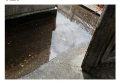
**Location:** Exterior Rear **System:** Exterior **Condition:** Water pools on walkway **Explanation:** The surface condition is such that there are dips in the walkway surface that may result in water pooling on the walkway.
