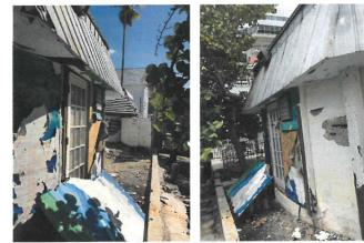
REMOVE ALL EXISTING DOORS AND ROOFING. REPAIR ALL CONCRETE SPALLING AT WALLS
