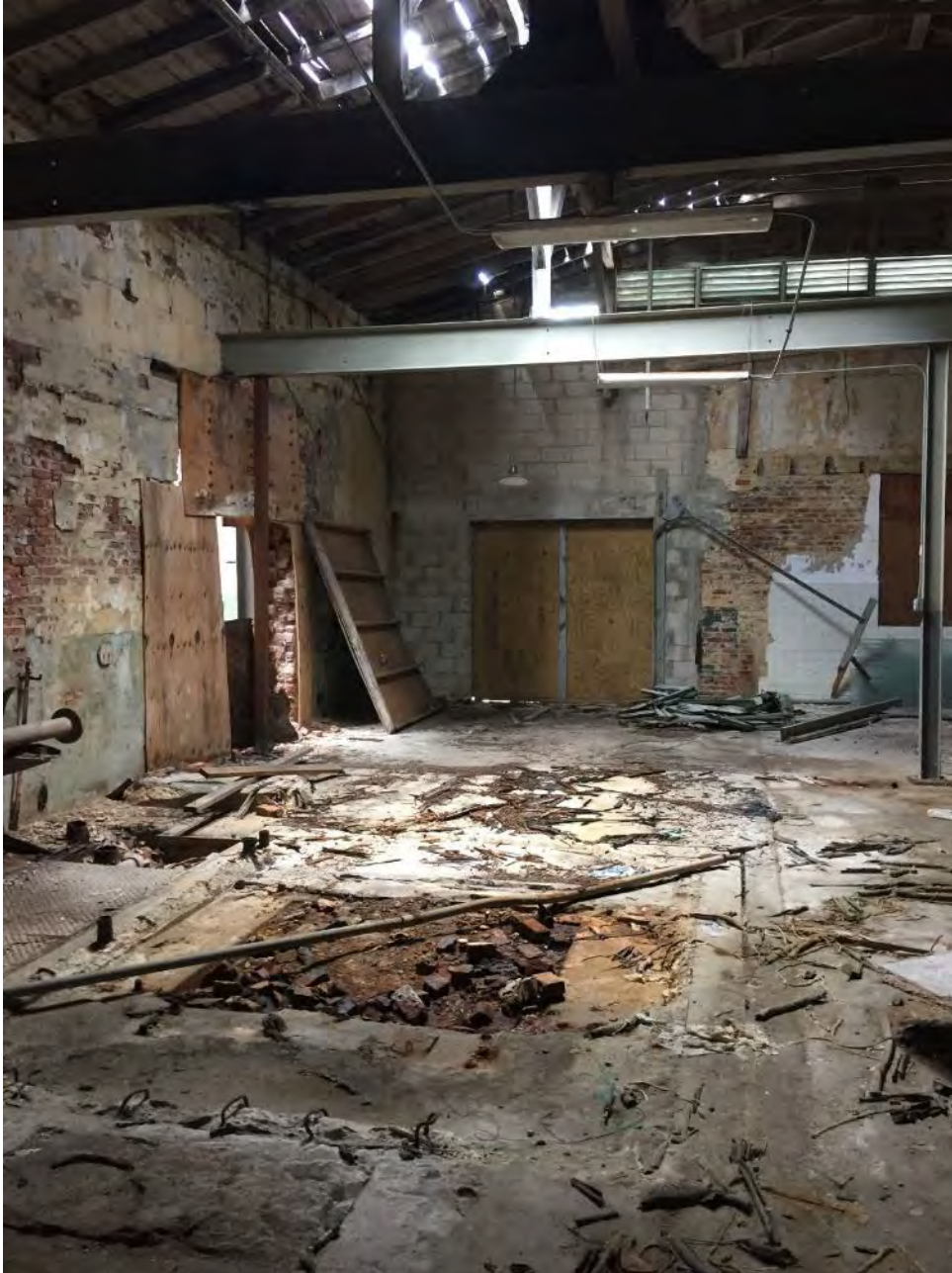
PHOTO 4: Interior of buildings at the Site
