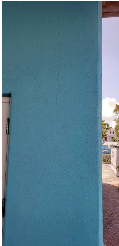
Figure 11. Location 9: Spalling cracks in the wall (corner tie-column).
