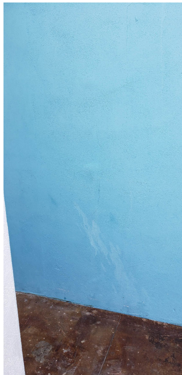
Figure 10. Location 8: Diagonal cracks in the wall developing here as well.
