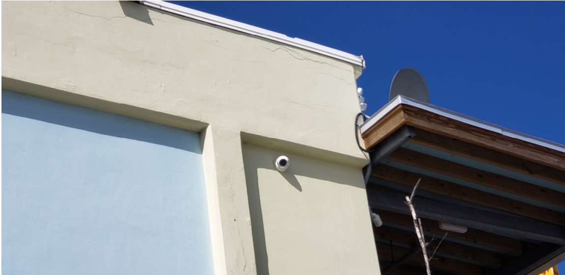
Figure 29. Between Location 20 and 22: The tie-beam has extensive cracking the top.
