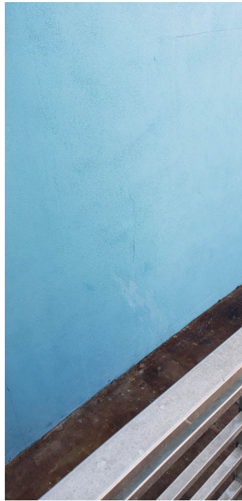
Figure 9. Location 7: Diagonal cracks in the wall developing
