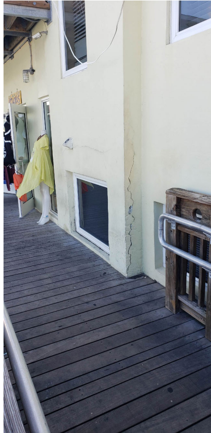
Figure 47. Location 40: Large cracks and heavy spalling of concrete in corner column.
