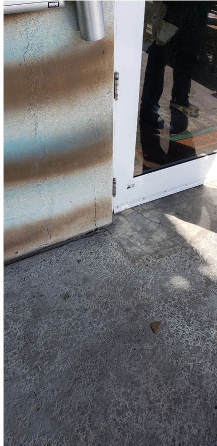
Figure 21. Front Entrance. Location14: Crack formation in the side of the opening.
