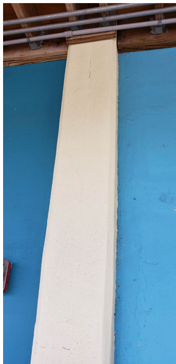
Figure 24. Location 17: Well developed cracks in the column center.
