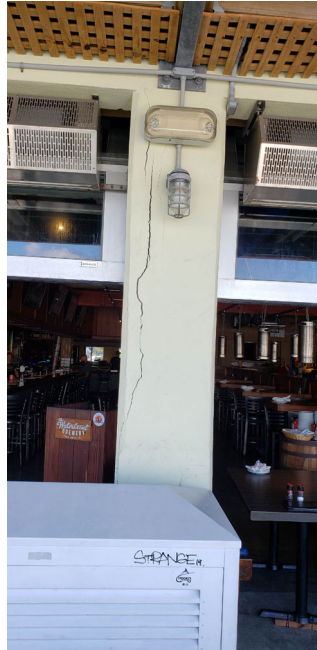
Figure 41. Location 34. Heavy damage in the column nearly next to entry to waterfront brewery from board walk side.
