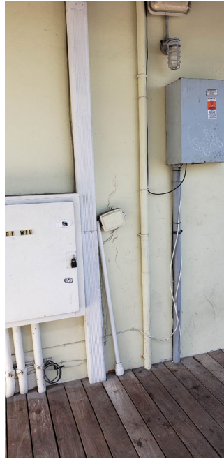
Figure 37. Location 30: Concrete spalling in the wall coupled with several cracks.
