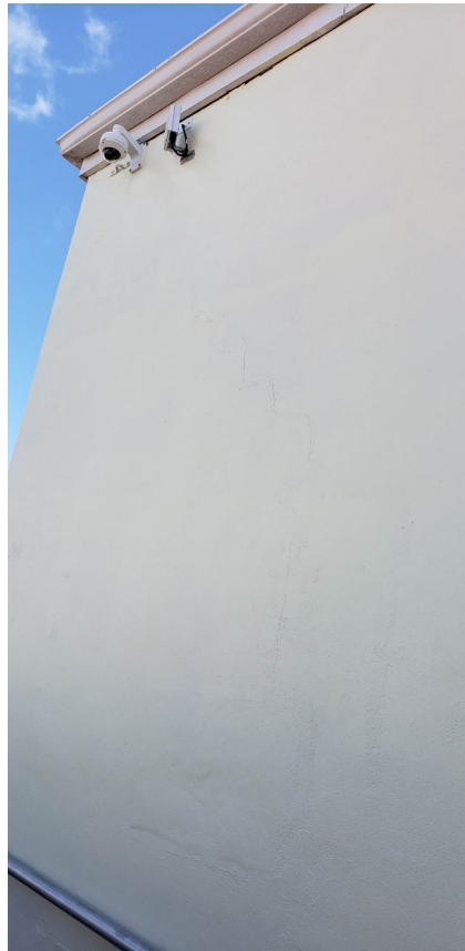
Figure 49. Location 42. Step ladder cracks visible propagating further down
