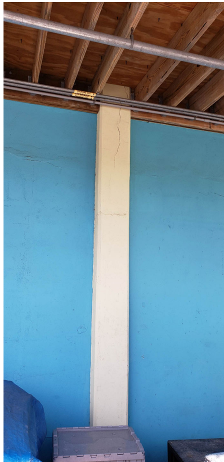
Figure 28. Location 19: Heavy cracking in the column at its mid-height approximately.
