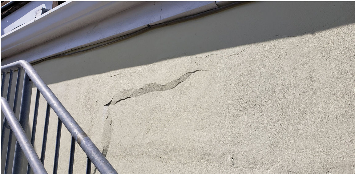
Figure 34. Between location 25 and 26. Above the staircase, the concrete tie-beam at the top has significant cracking in it. Heavy spalling and delamination of the concrete
