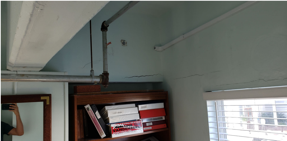
Figure 53. Location 44: The tie-beam above the window on the second floor at location 44 is getting large horizontal cracks.
