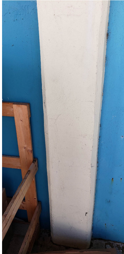
Figure 25. Location 18: Developed spalling cracks in the bottom of column.
