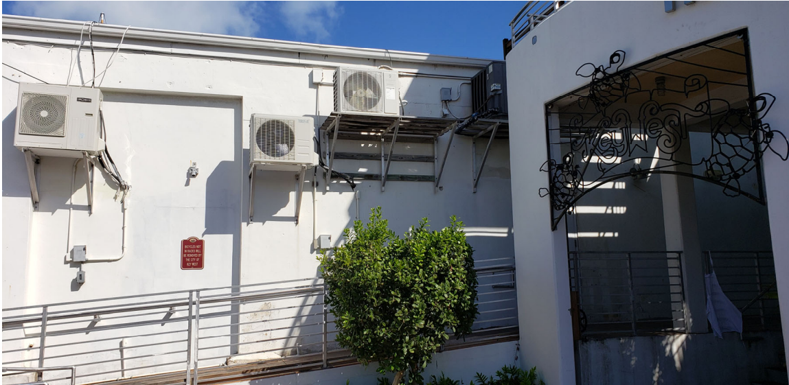
Figure 5. Front Elevation near roundabout. Location 4: Horizontal tie-beam cracks seen near the AC units. Vertical cracks at the top of the CMU wall also develop above the horizontal cracks in the tie-beam.
