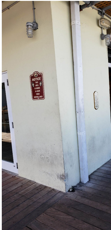
Figure 38. Location 31: Corner of the column showing concrete spalling covered with paint and sealant.
