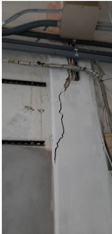
Figure 6. Interior of the Building. Location 4: The interior portion of the column is heavily cracked. Large diagonal cracks along with concrete spalling is observed. Existing electrical conduit is supported to a pipe sitting in the damaged portion.
