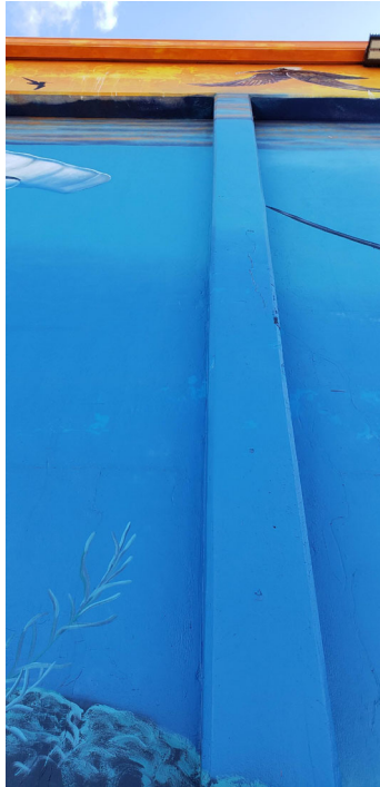
Figure 15. Location 11: Heavy cracking and spalling in the column. Please note that some of the cracks are not as obvious since they are covered by elastomeric paint and sometimes sealant.
