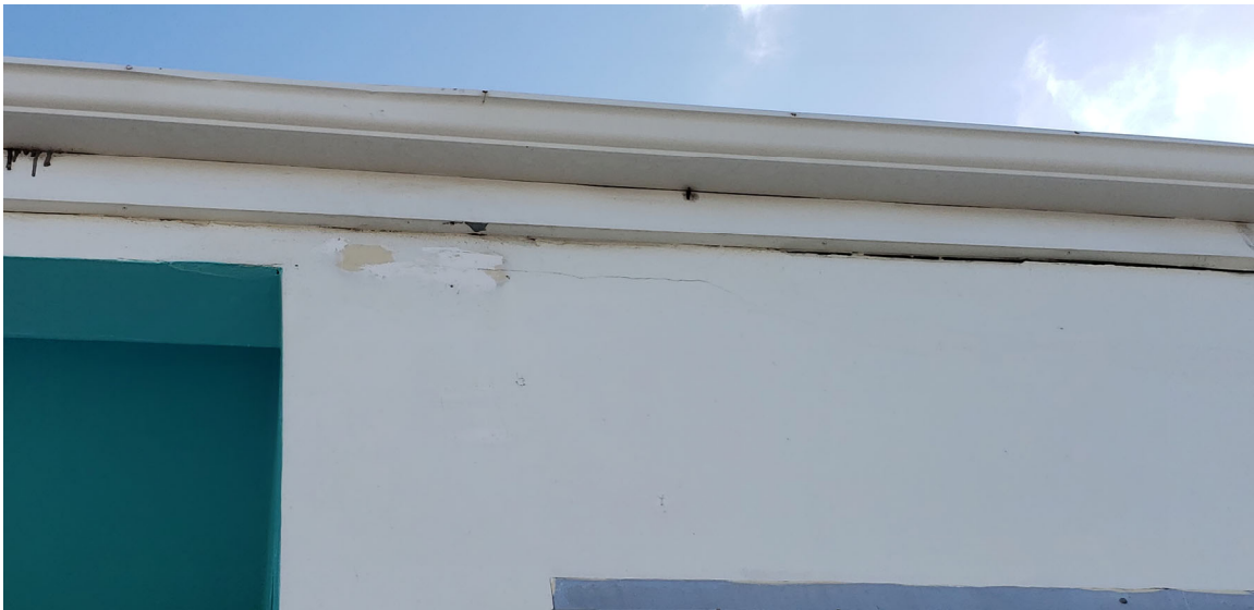
Figure 50. Location 43: Cracks forming in the wall at roof level. Please note that top of roof level tie-beam is concealed with fascia board and gutters. Likely more similar spalling will be observed.
