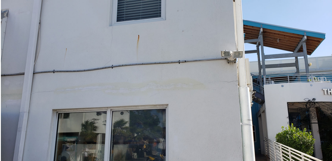
Figure 52. Location 44: Cracking in the tie-beam is continued here from Figure 50 as well. The portion of the wall above the tie-beam is also experiencing vertical cracking (bottom left corner of the top window).
