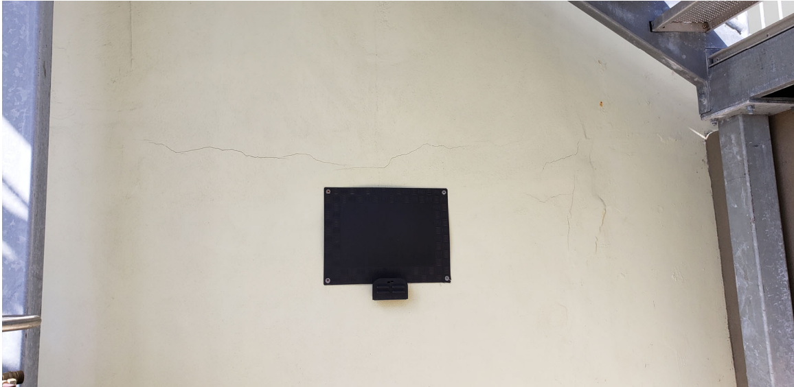
Figure 35. Location 28: Cracks formed in the wall in this area underneath the staircase as well.
