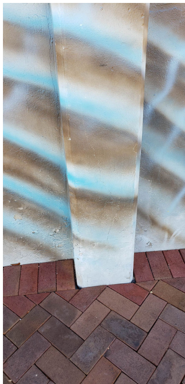
Figure 14. Location 10: Cracking in the column consistent with progressive spalling.
