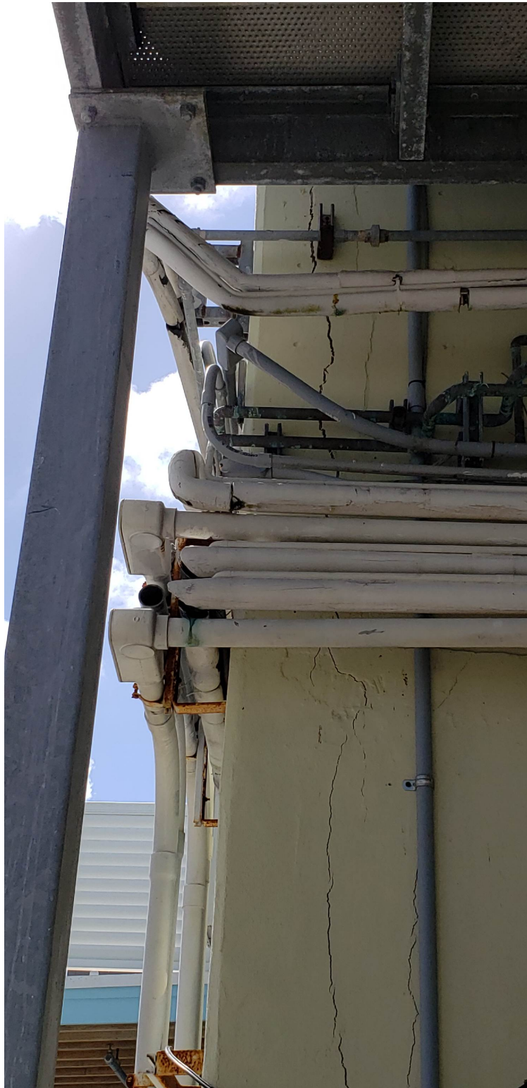
Figure 31. Location 22&23: Same as location 21. Heavy damage of the concrete corner and wall.
