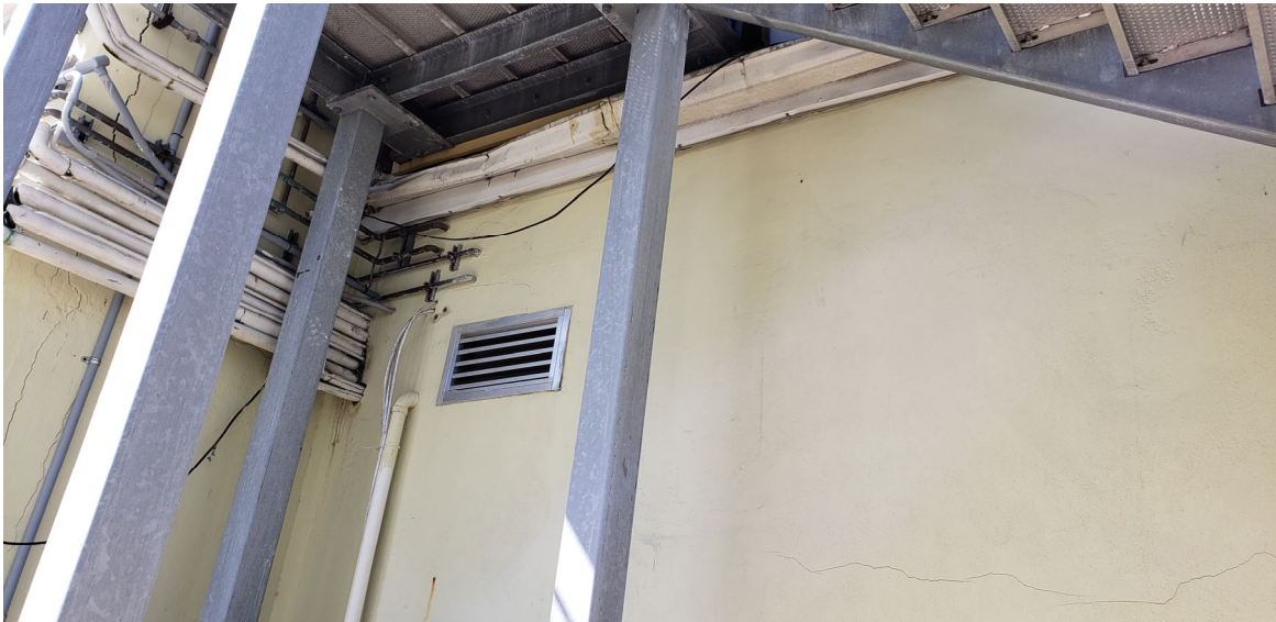
Figure 33. Location 25: Cracks in the wall (likely horizontal tie-beam spalling).
