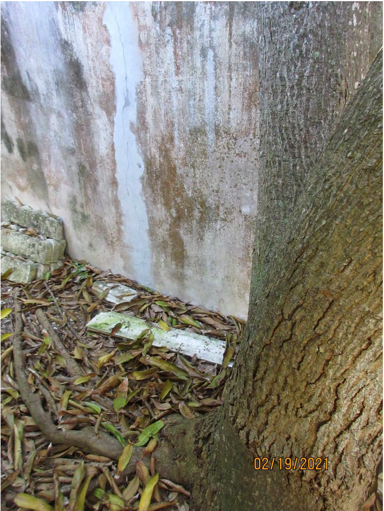
Photo showing base of tree and cracks in wall.
