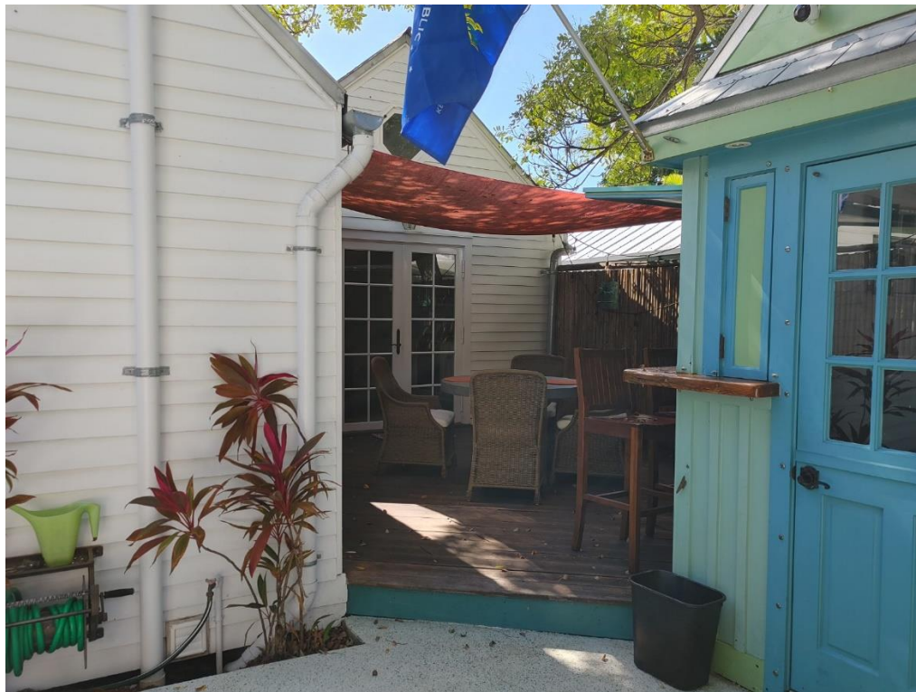
Subject deck area
