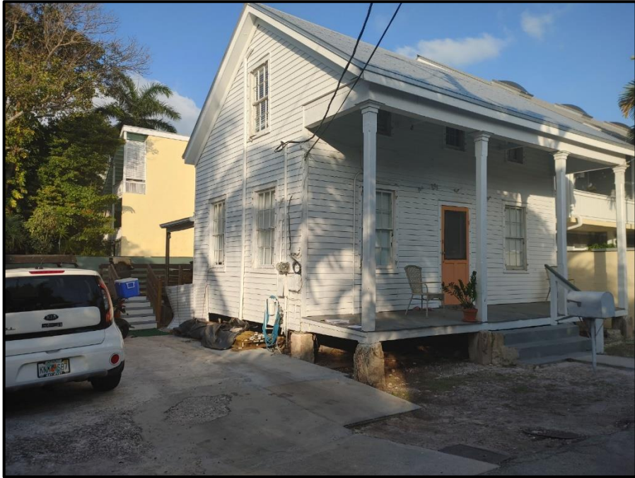
608 Griffin Lane – Site visit on March 24, 2021
