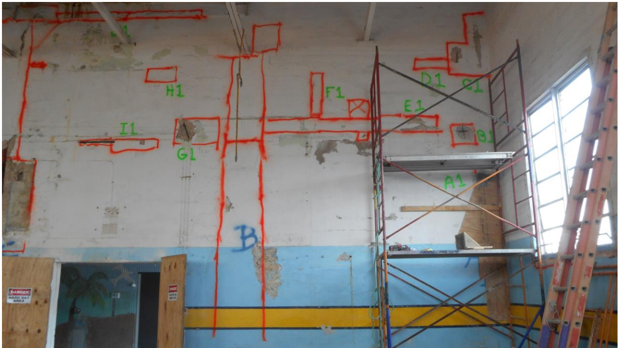
Spalling Repair at Historic Glynn Archer Gymnasium, Key West
