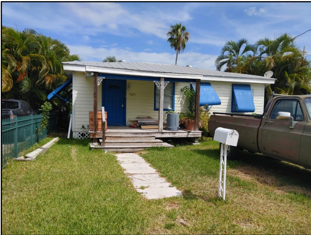
2827 Harris Avenue existing one-story structure
