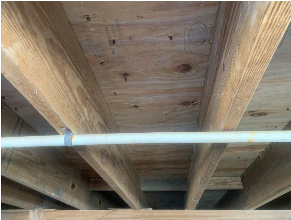
Existing floor framing under original historic house – 100% replaced in 1990's renovation with exception of perimeter sill beam
