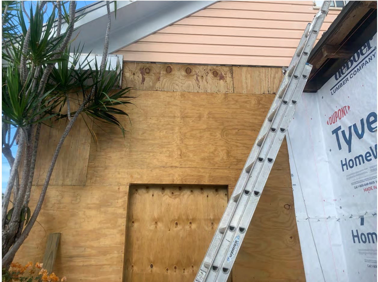
Rear wall of original historic structure – current front door location Plywood and siding at gable from 1990's renovation New exterior plywood added below gable to make lower wall flush with gable wall above
