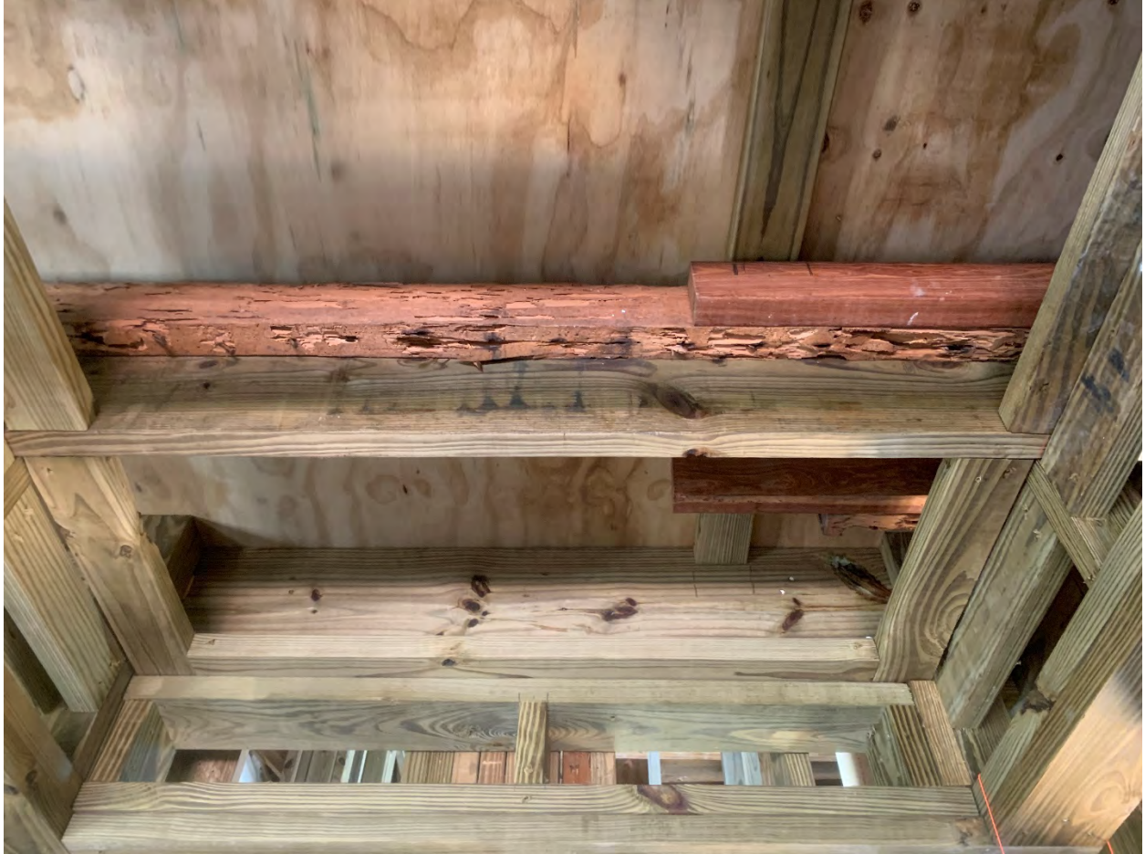
Example of damaged ceiling joist at rear addition Plywood is attic floor above from 1990's renovation
