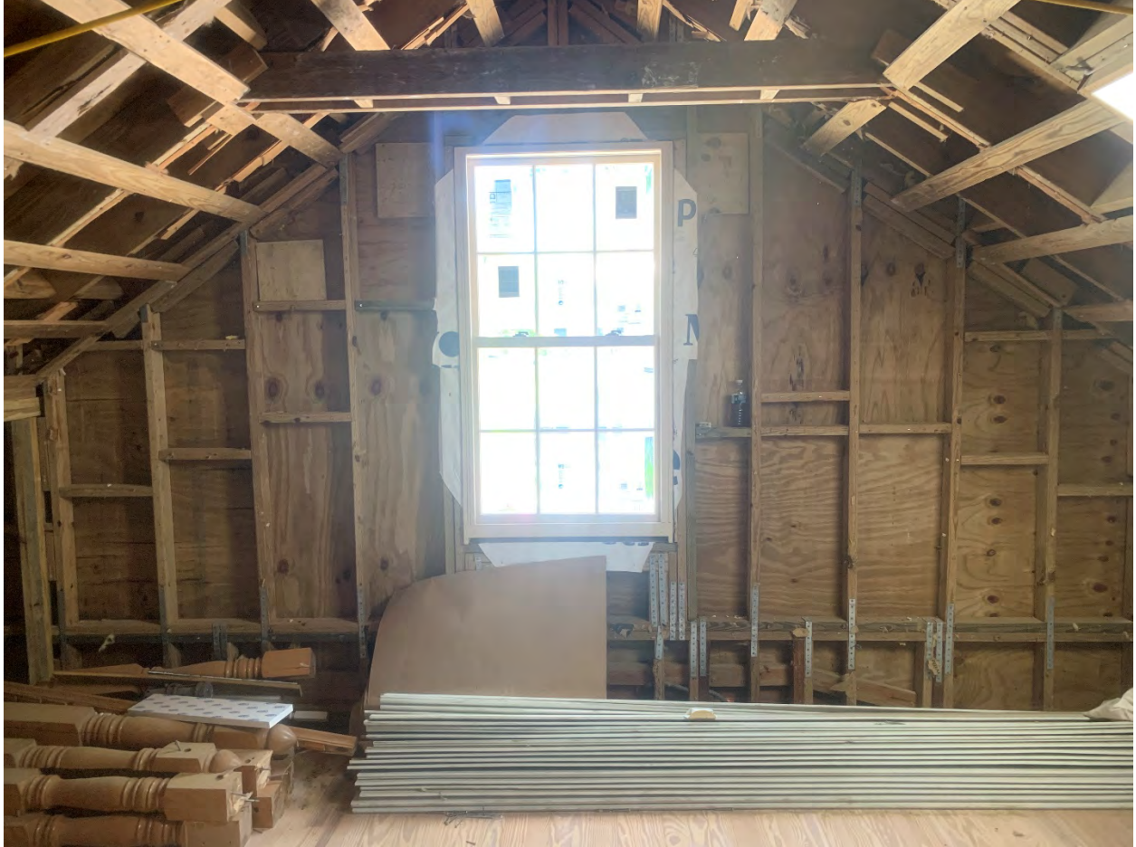
Inside of original historic structure front wall at 2 nd Floor Framing and exterior plywood sheathing from 1990's renovation Sistered rafters from 1990's renovation New larger window (for emergency egress) was properly permitted
