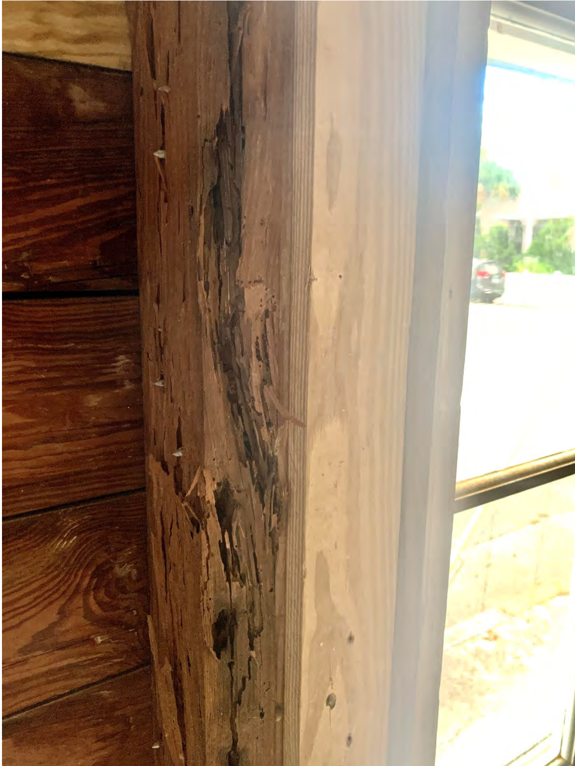
Example of damaged historic wall stud at South Wall facing Pine Street
