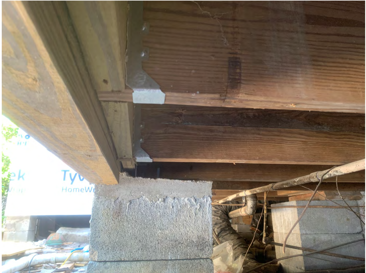
New concrete pier and sill beam at north wall of historic house Floor framing from 1990's renovation
