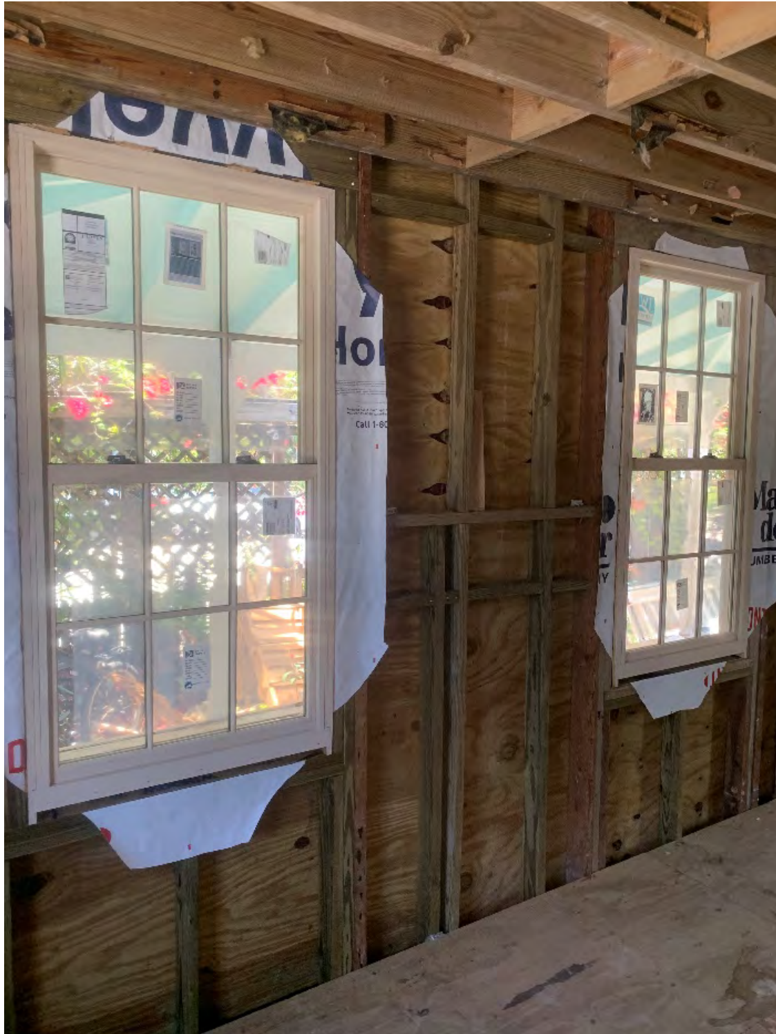
Inside of Historic Front Wall facing Georgia Street New exterior plywood sheathing Sistered wall studs and 2 nd Floor Framing (ceiling) from 1990's renovation
