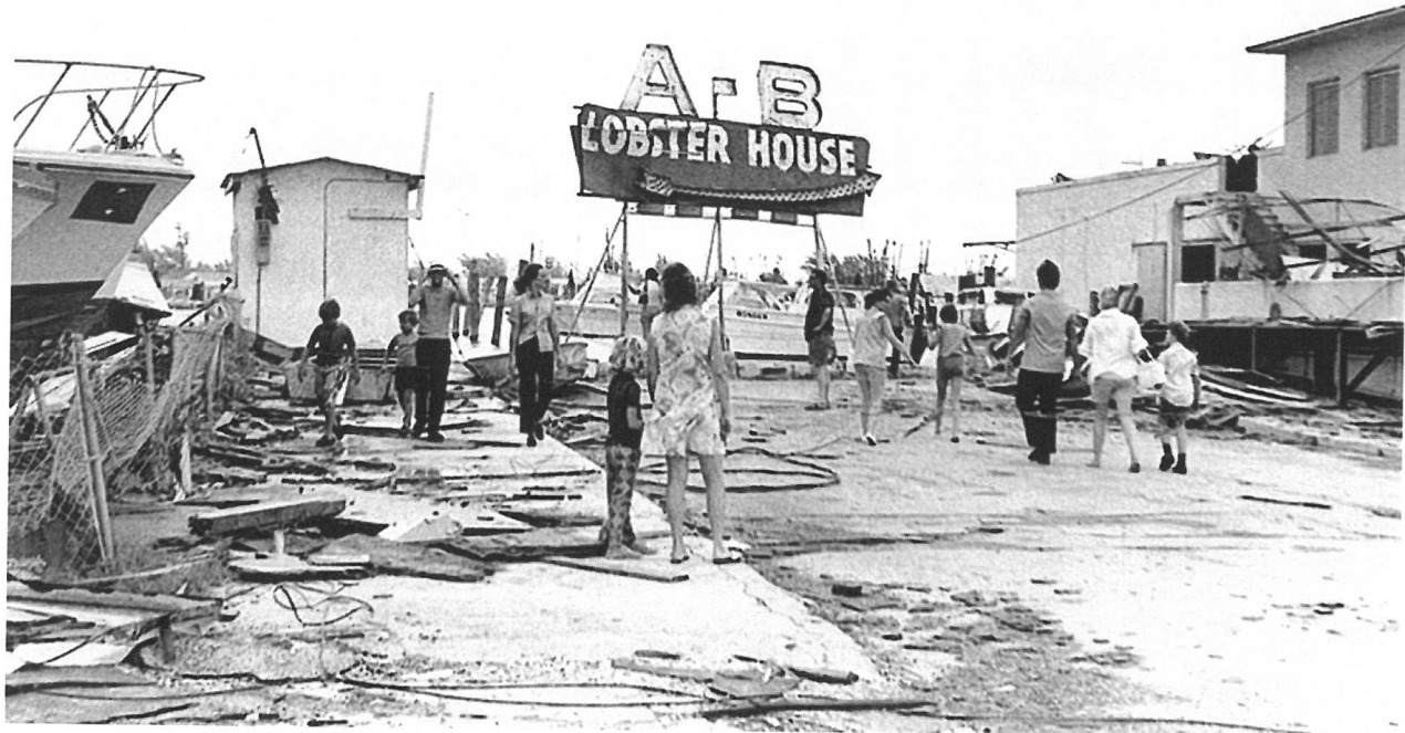
*A&B sign and building still standing following devastating tornado from Hurricane Agnes in 1972
