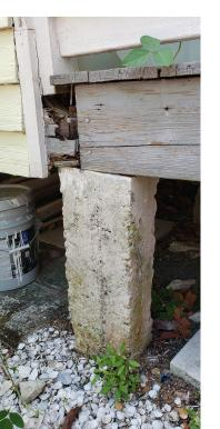
Support beams rotting on unstable piers, large boulder holding corner up.
