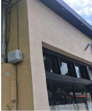
2018 Storefront: Replaced & redesigned storefront, new concrete columns & façade.
