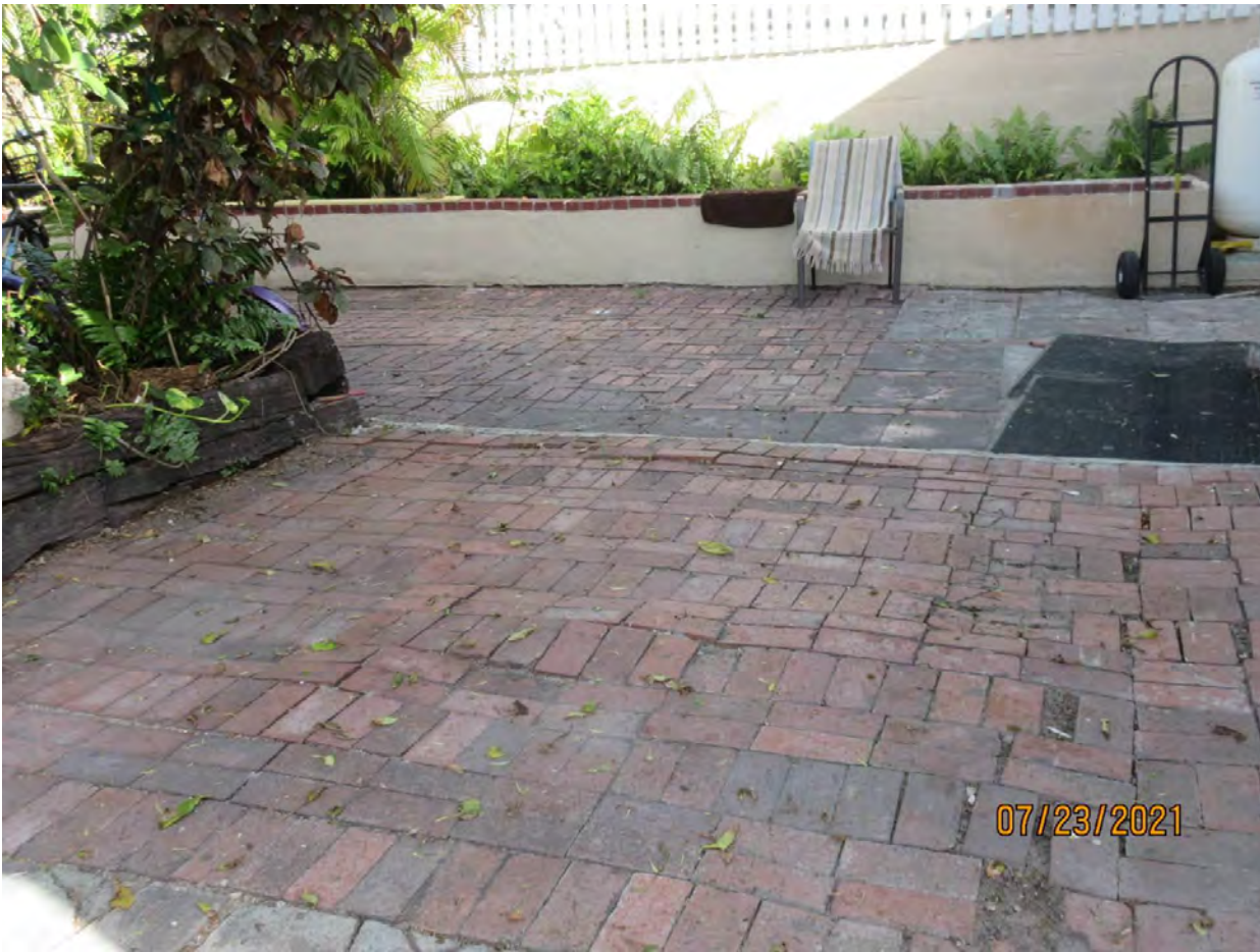
Photo of adjacent paver area and root impacts, view 1.
