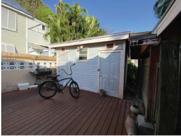
EXISTING ACCESSORY STRUCTURE
