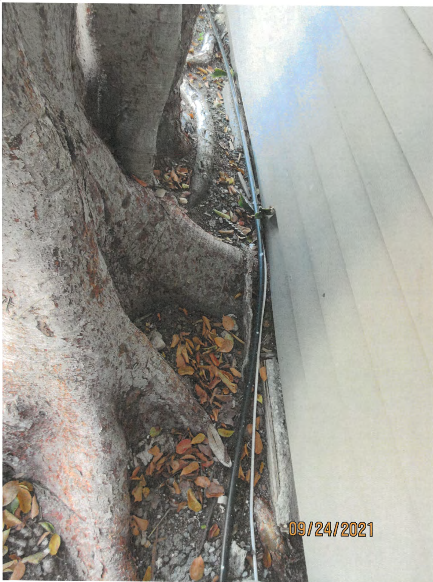
Photo showing tree roots growing under structure. KCD
