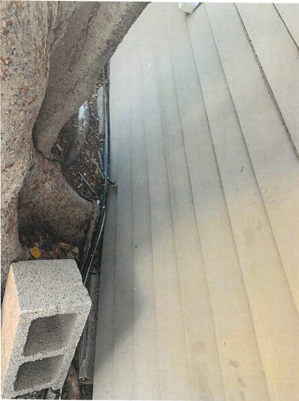
photo showing tree roots growing under structure. RD
