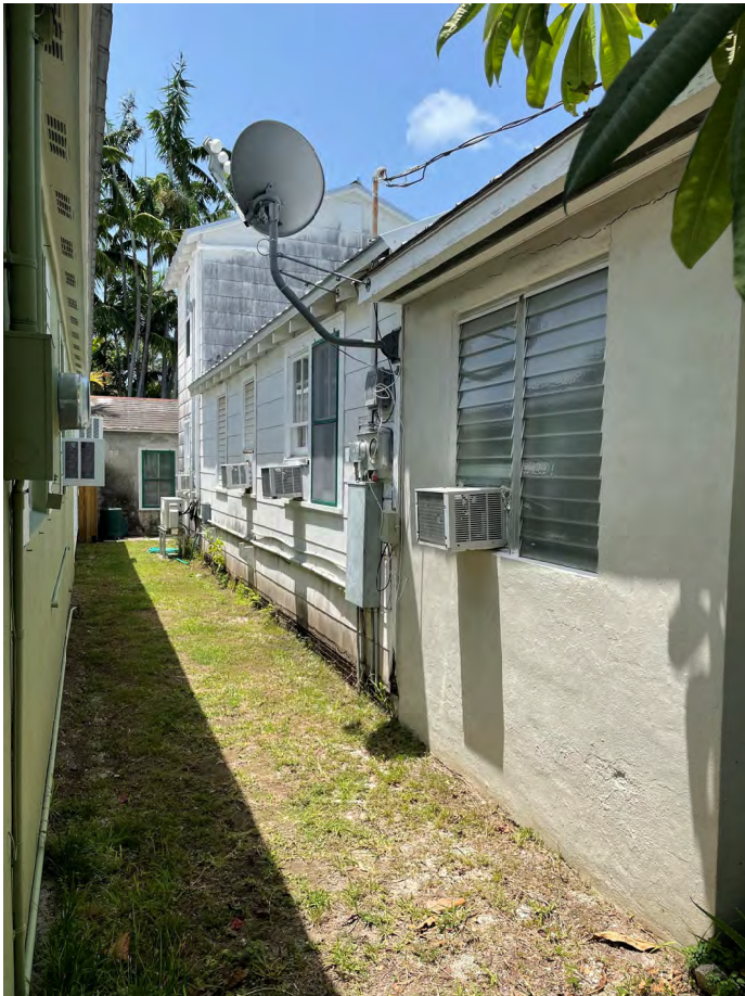
Existing Left Side of House – 1108 Grinnell
