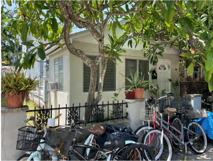
Existing Front of House – 1108 Grinnell
