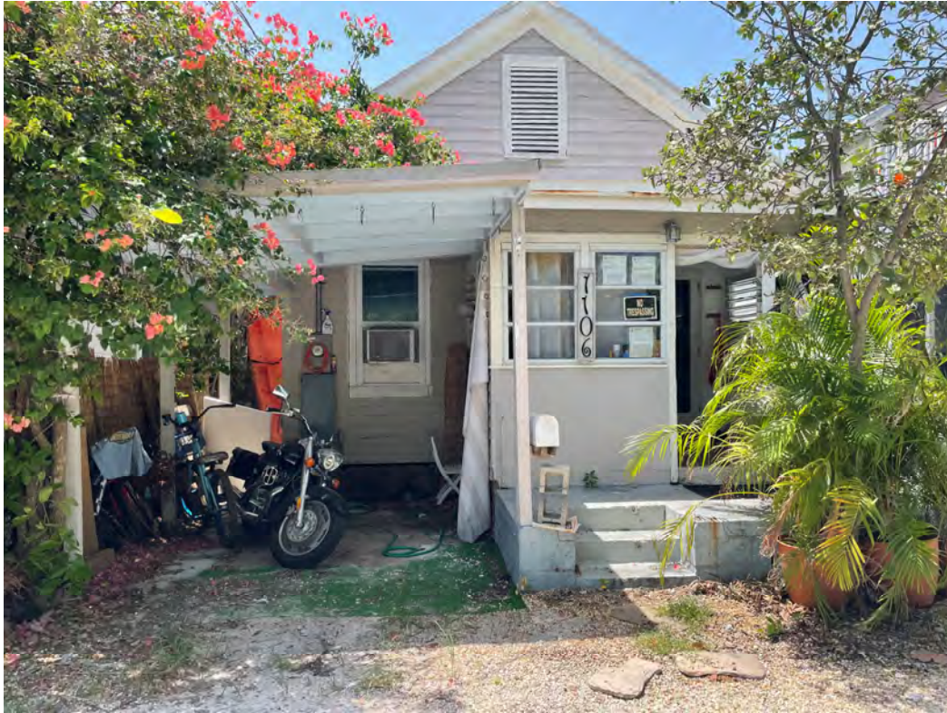
Adjacent Property to North
