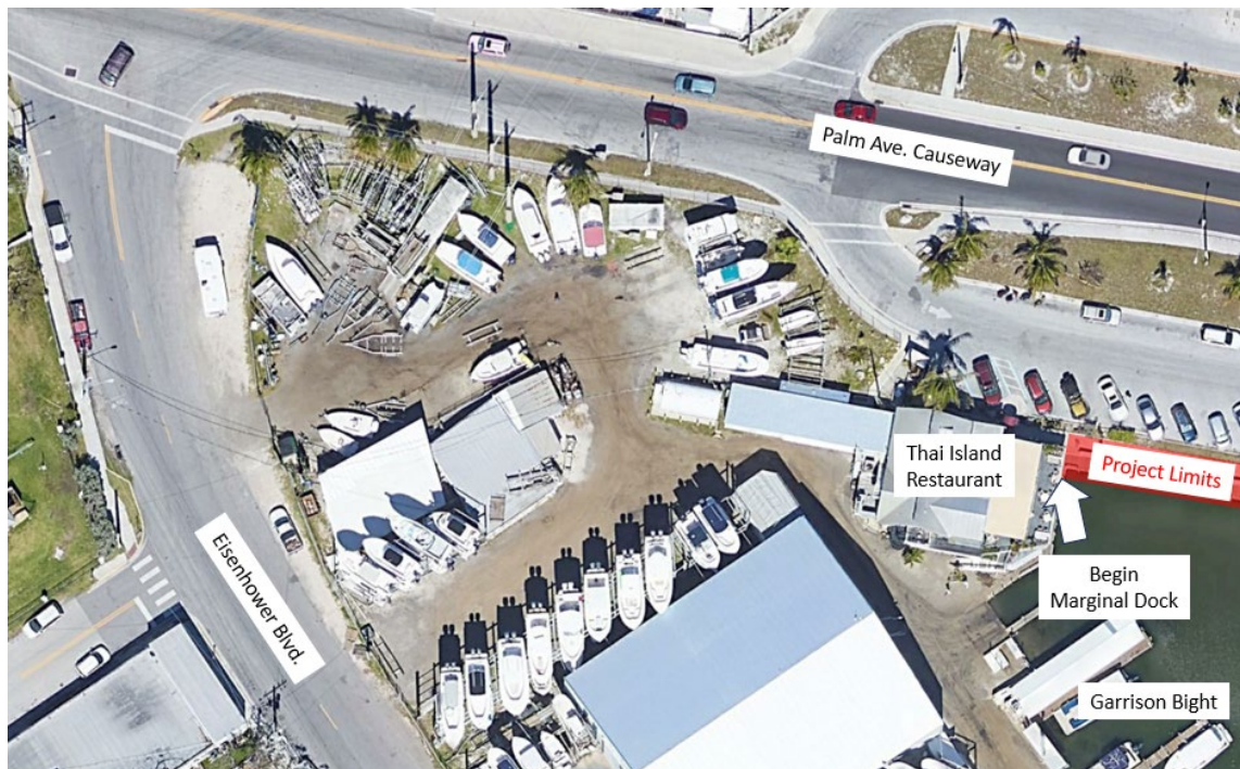
Insert 2: Western Limits of Seawall Replacement, and Eisenhower Blvd for Utility Sourcing
