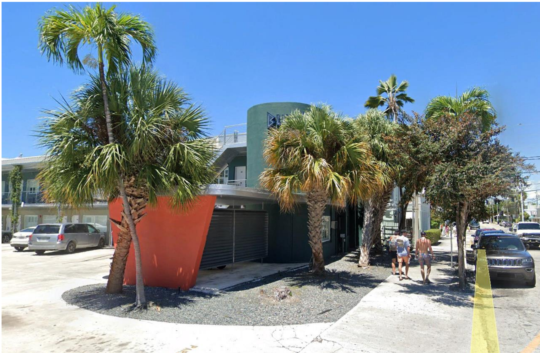
1314 Simonton Street, Key West, Florida 33040 SITE VISIT
