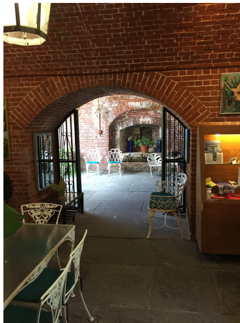
8' Back Door to be Replaced
