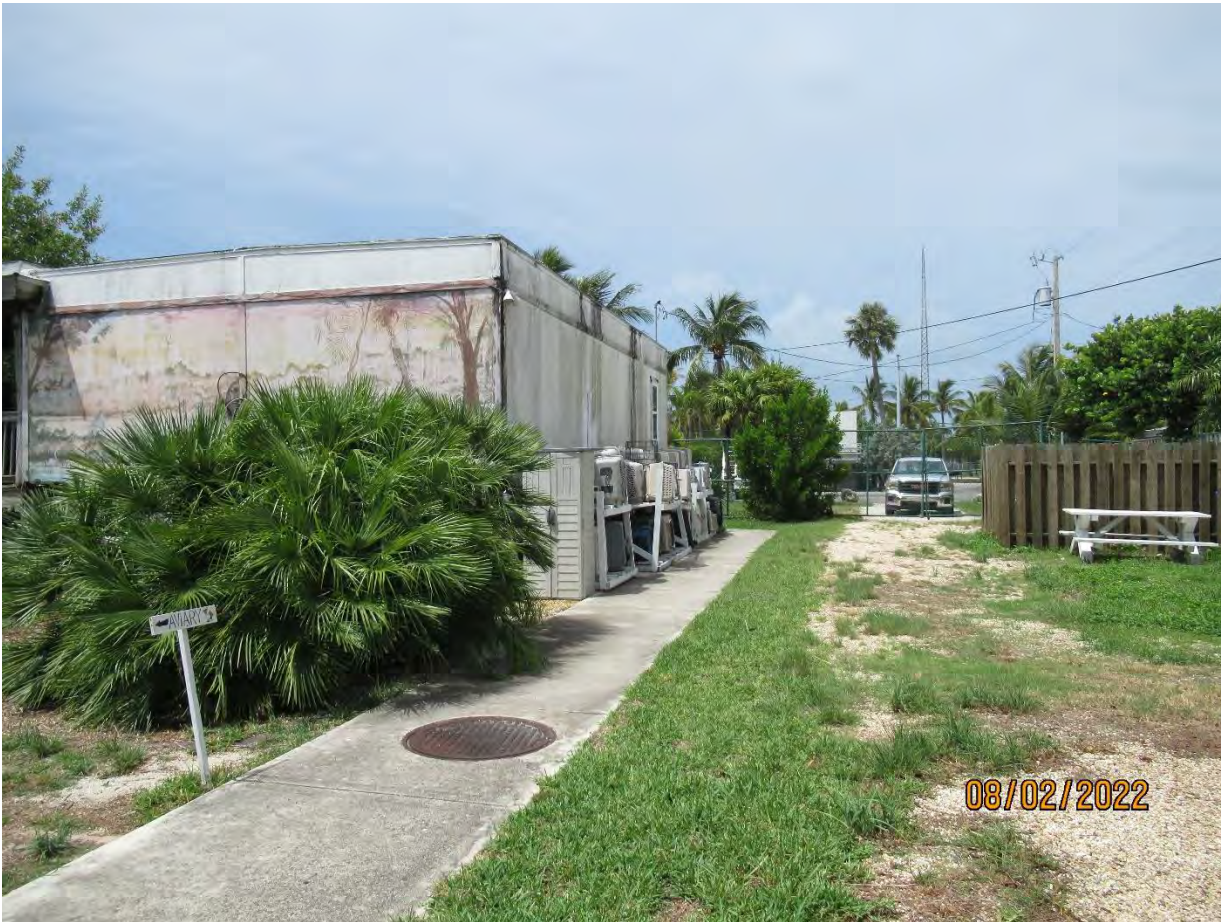
Standing at the northeast corner of the proposed work area looking to the west, view 2. New building to be constructed in front of existing structure.
