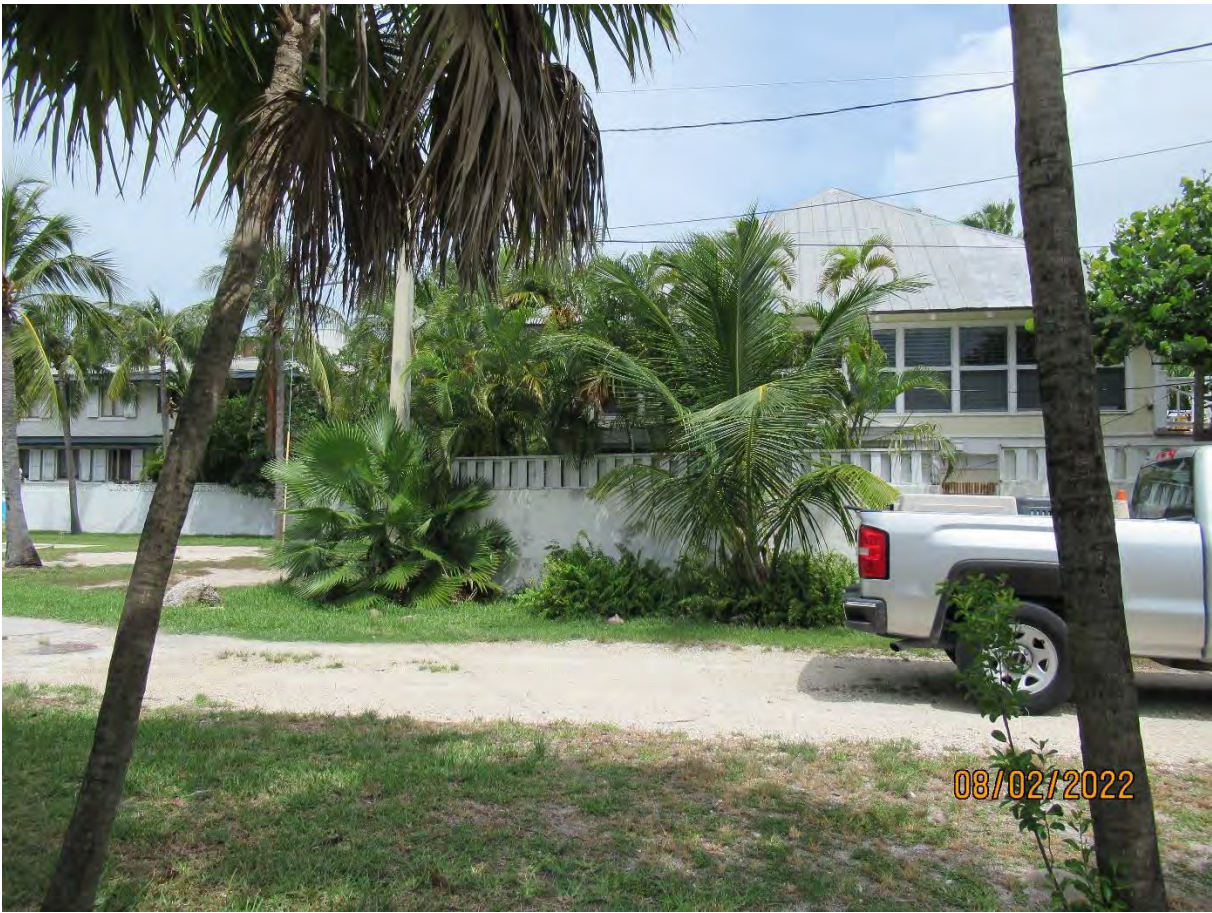
Photo of northern property line area. Palms to remain in place and be protected.
