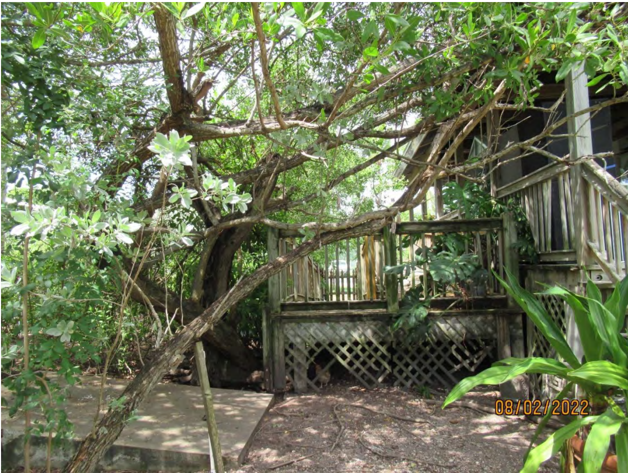
Photo looking west at the south side of the existing structure, area will need to be properly trimmed prior to construction and demo work.
