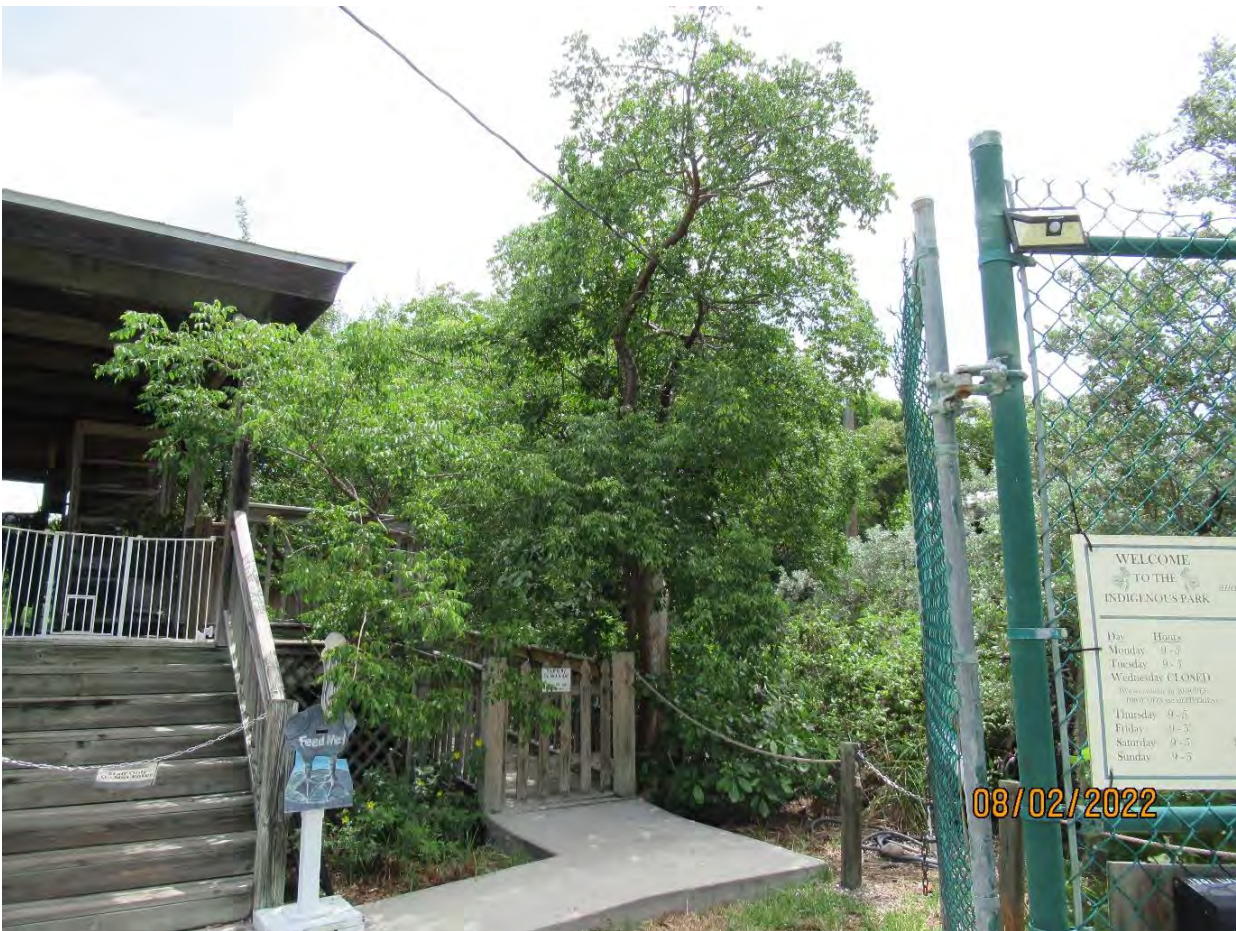
Looking east, existing structure to demolished once new structure completed. Tree #13 & #16- Gumbo Limbos, to be transplanted.
