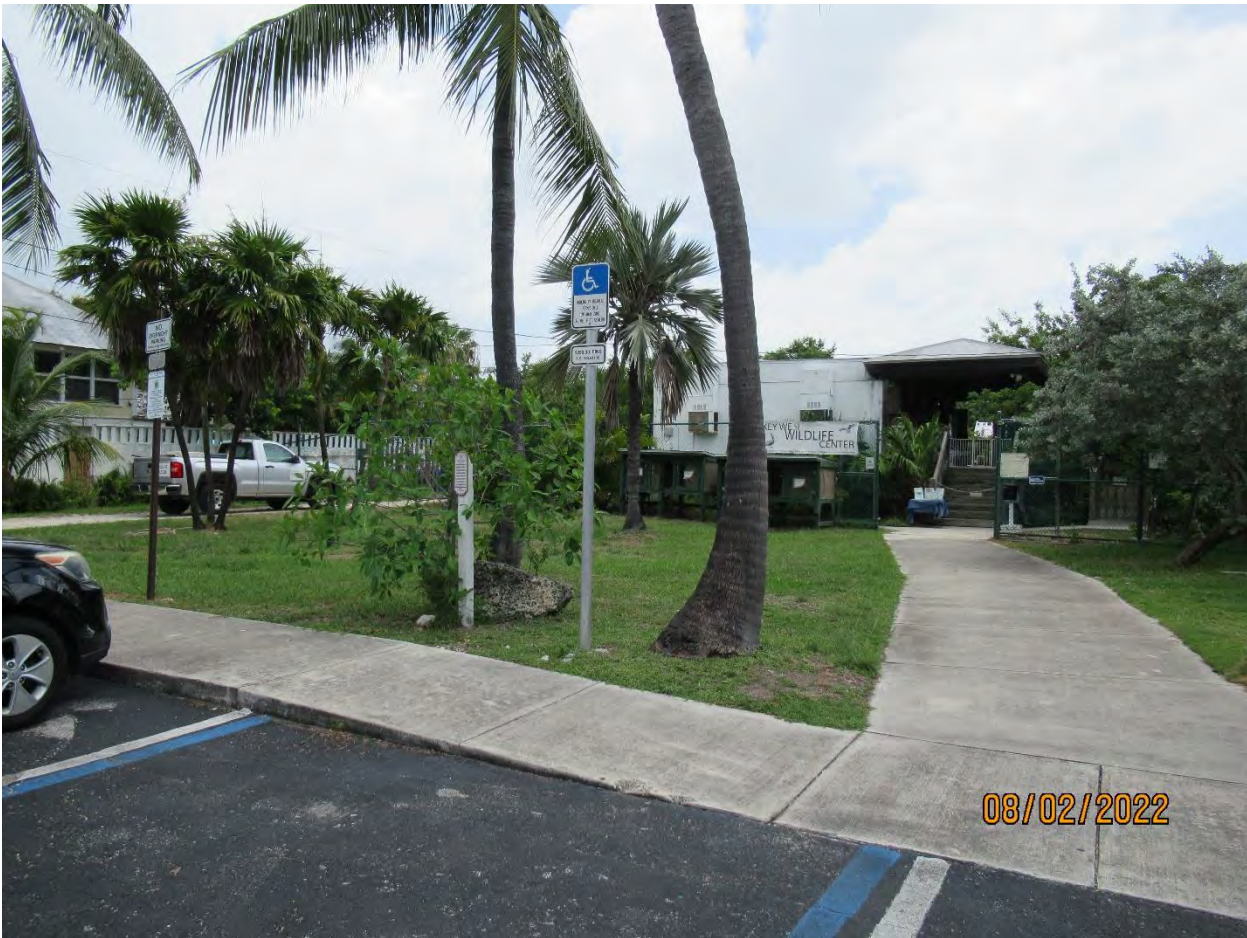
Looking toward the east at the proposed work area, trees #17, #2, #7, and #4 to be transplanted. Coconut palm nearest sidewalk to remain and be protected.
