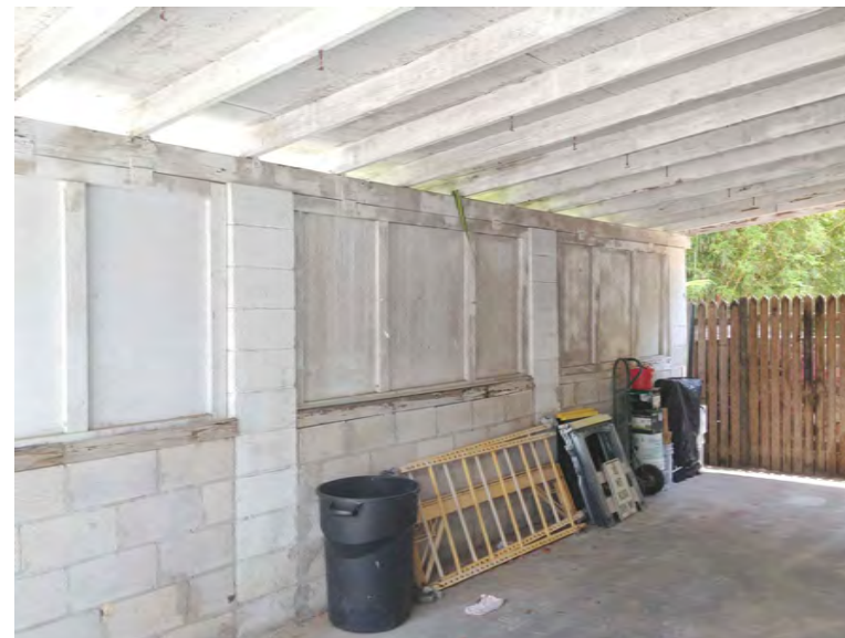
FIGURE 5 INTERIOR VIEW OF CAR PORT
