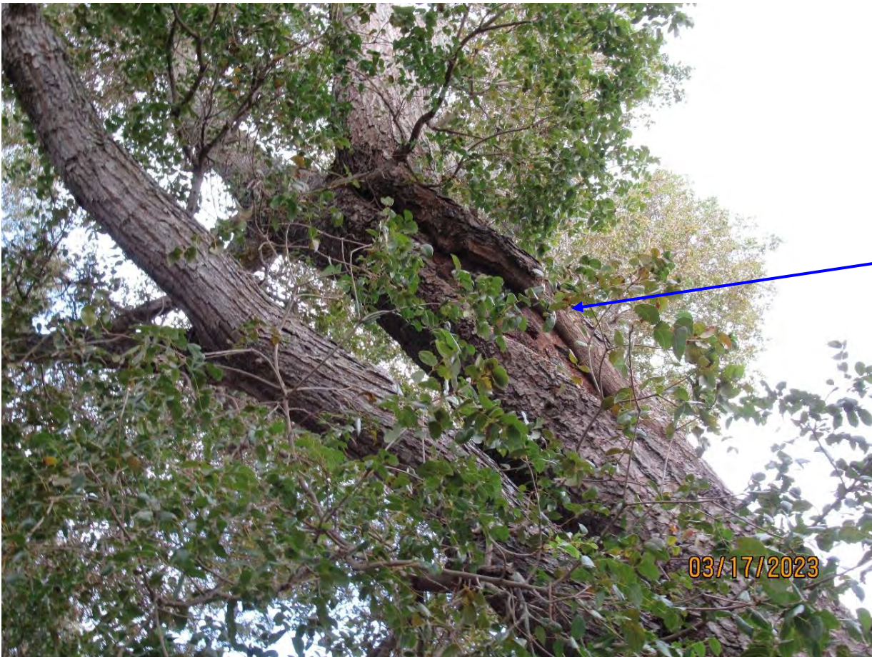
Large decay area in main canopy branch/trunk.
