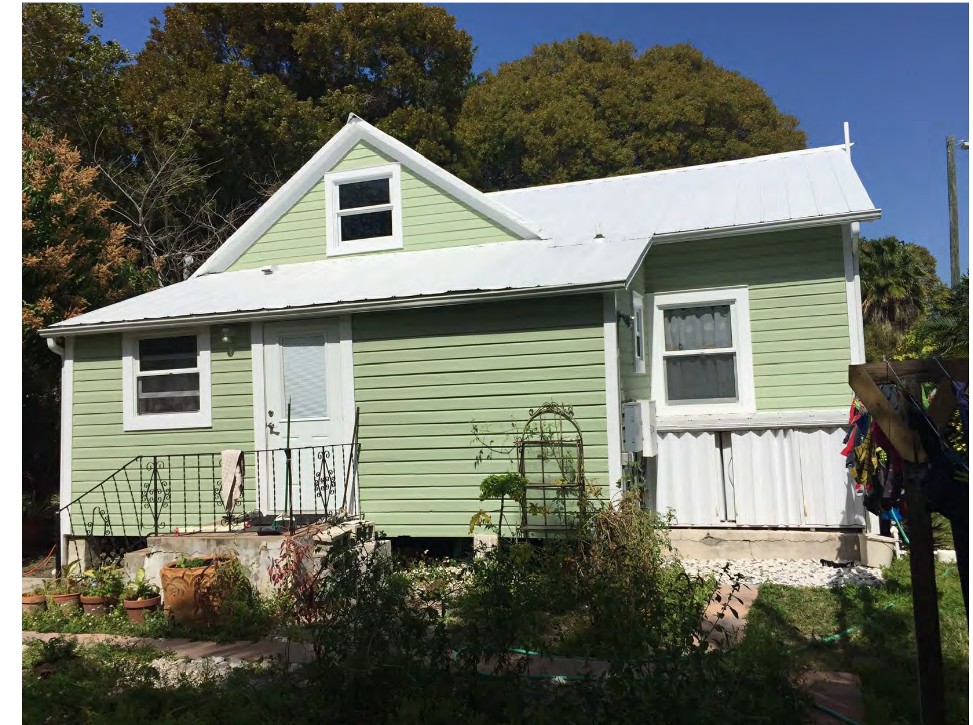
PHOTO OF WEST FACADE (REAR YARD)
