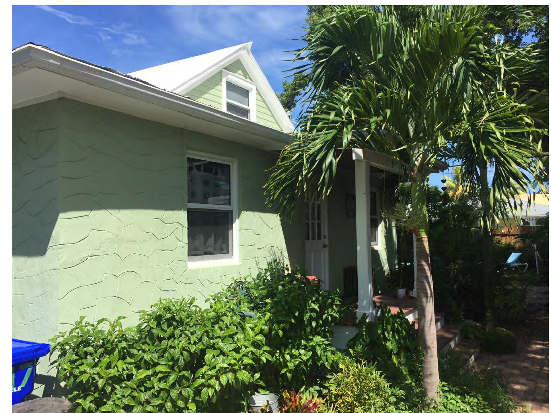
PHOTO OF GEORGIA STREET FACADE (EAST FACADE)
