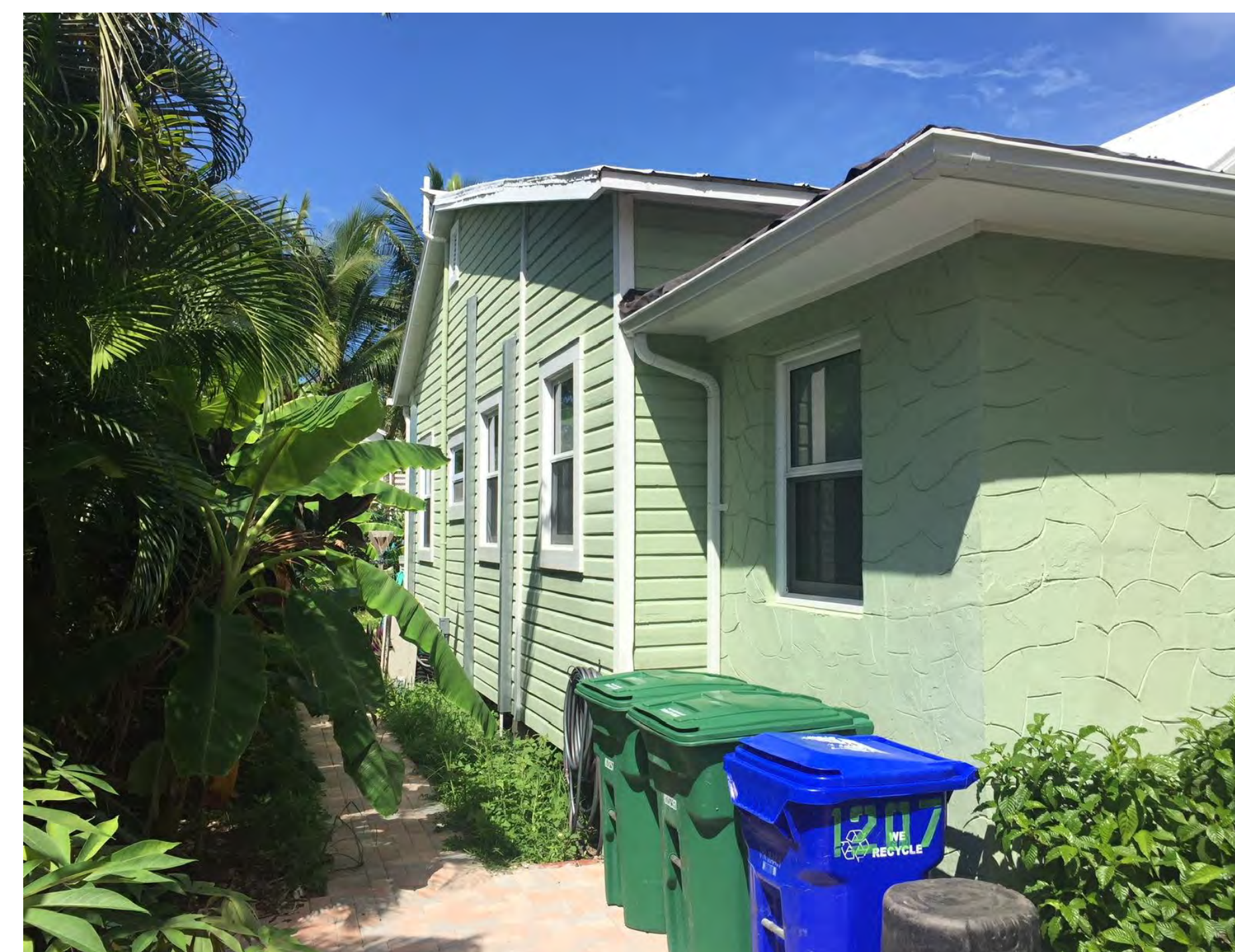
PHOTO OF SOUTH FACADE
