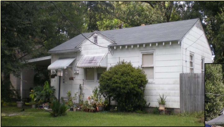
(DU20489) 1182 Scotten Street
