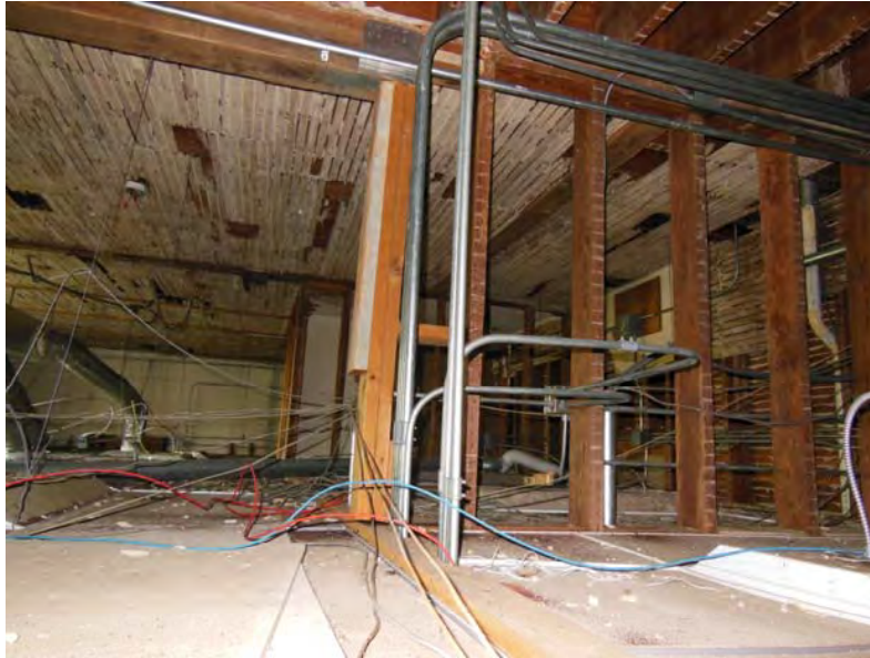
#9 Building A Existing Condition: Roof Framing
