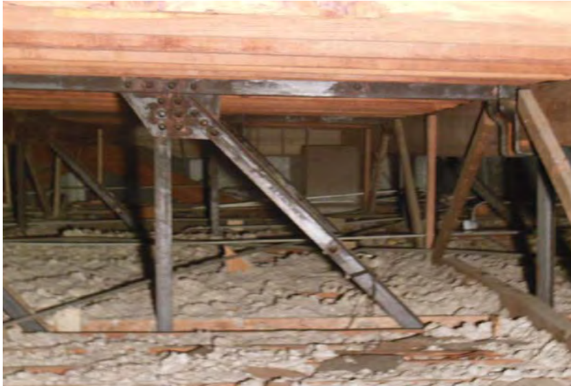
#5 Auditorium Roof Framing Existing Condition: Steel Truss Framing East-West Direction
