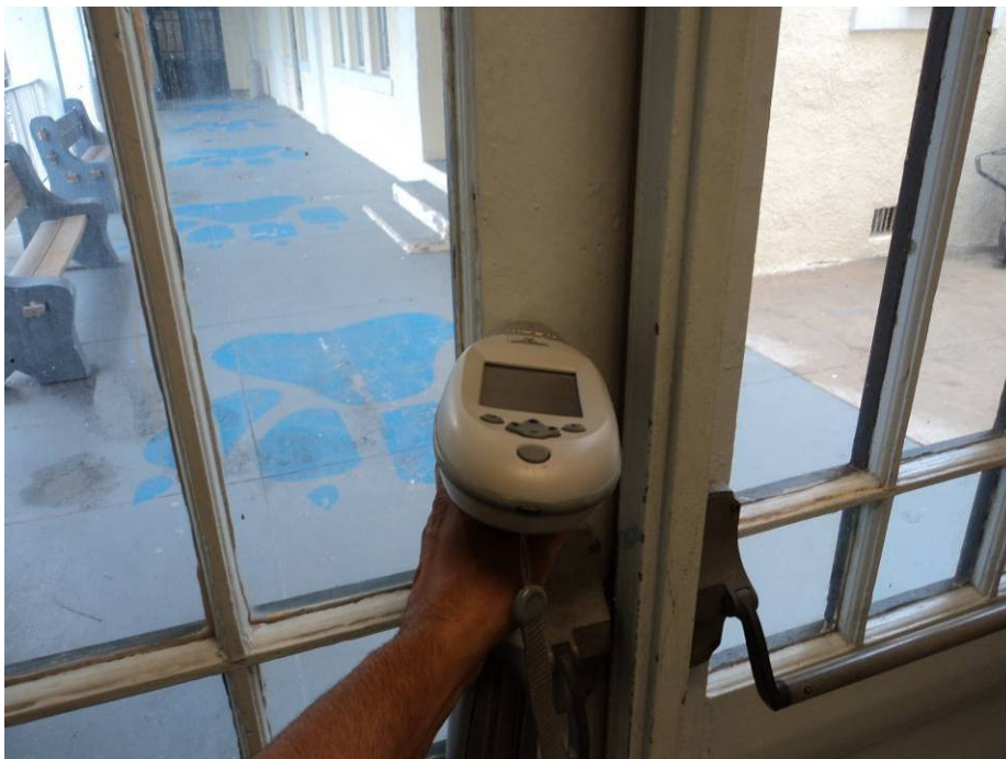
Photograph #10: Typical wood door identified with LBP during this inspection (XRF #196, 219, 220).
