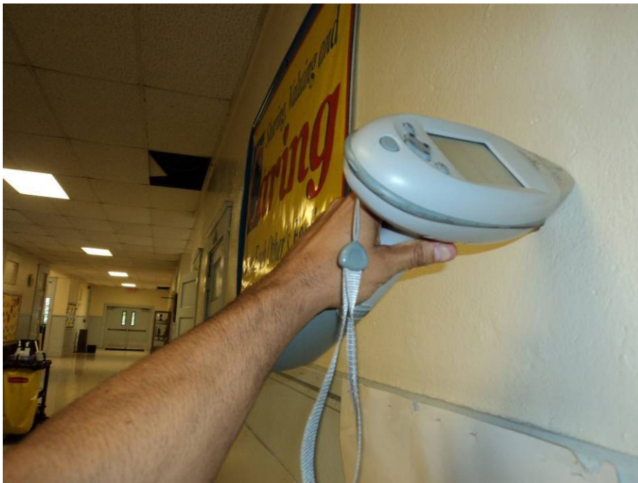
Photograph #4: Wall paint identified with LBP (XRF #43).
