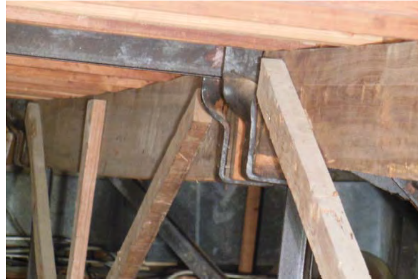
#6 Auditorium Roof Framing Existing Condition: Wood Truss Framing North-South Direction
