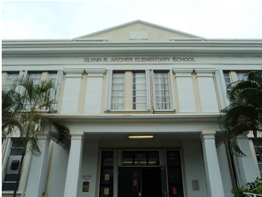
Photograph #23: Front entrance to Glynn R. Archer elementary school.
