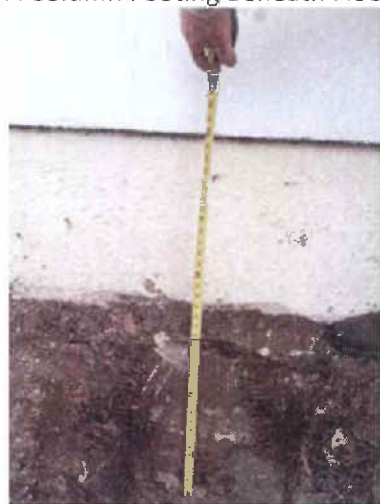
Building A East Wall Footing at NE Corner of Building
