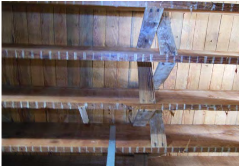
#11 Building A Existing Condition: Second Floor Framing Wood Joists
