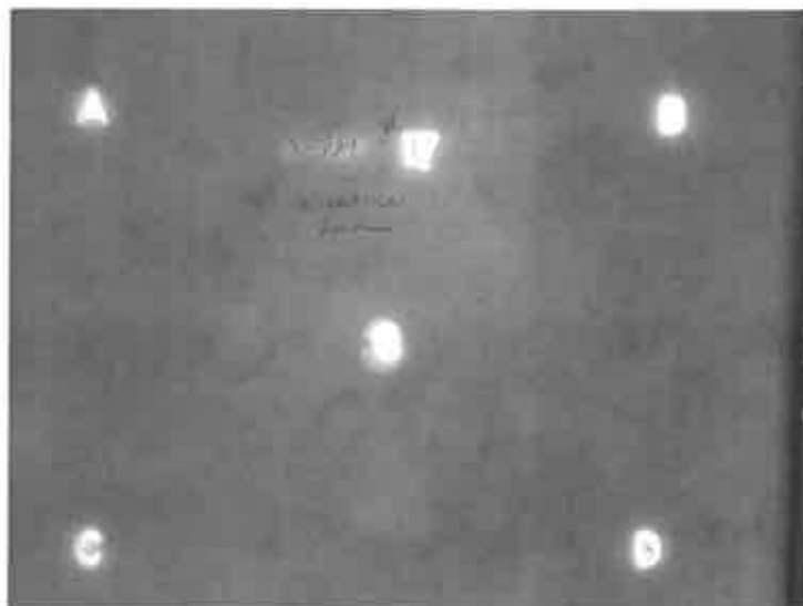
Electrical Room, West Side of Stage, West Corner – X-Ray # 17 & 18
