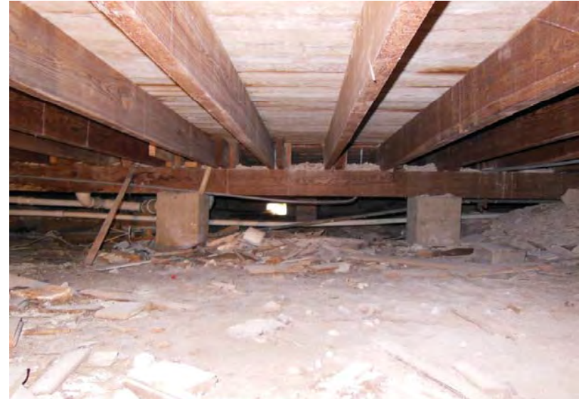
#2 Auditorium Foundation Existing Condition: Ground Floor Framing
