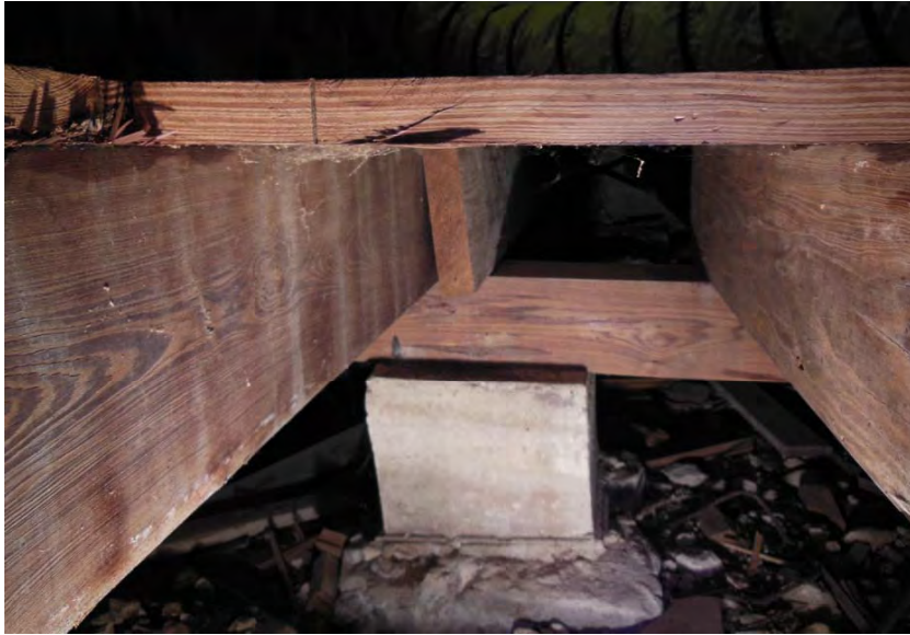
#1 Auditorium Foundation Existing Condition: Interior Spread Footing and Pier
