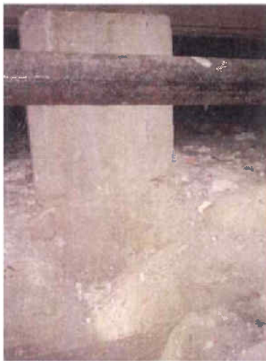
Building A Column Footing Beneath Floor System
