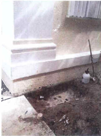
Building B South Wall Footing at SW Corner of Building
