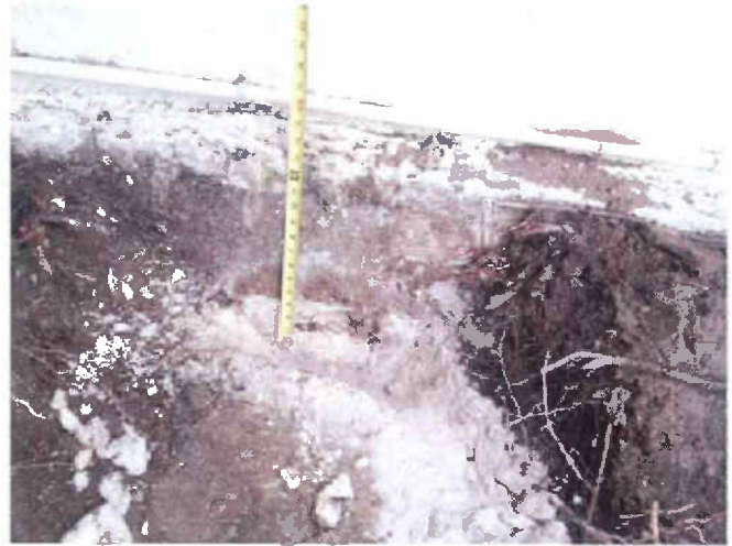
Building A North Wall Footing at NW Corner of Building
