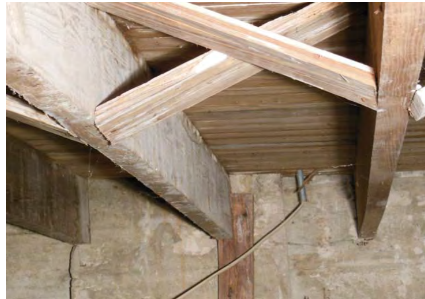
#8 Auditorium Perimeter Wall Existing Condition: Load Bearing Walls
