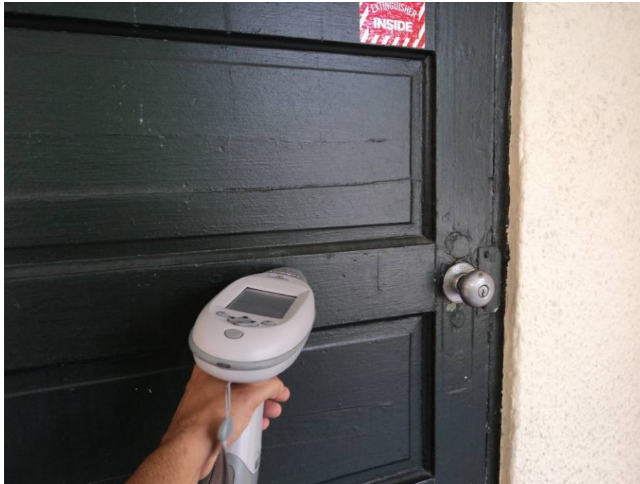
Photograph #21: Exterior door paint identified with LBP during this (XRF #504)
