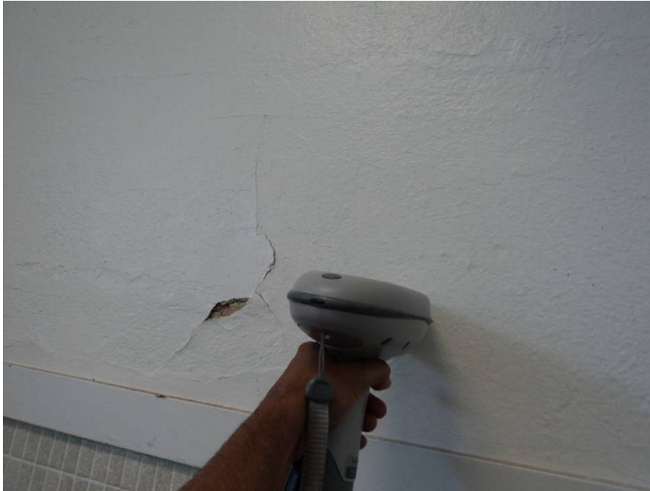
Photograph #1: Wall paint identified with LBP (XRF #15).
