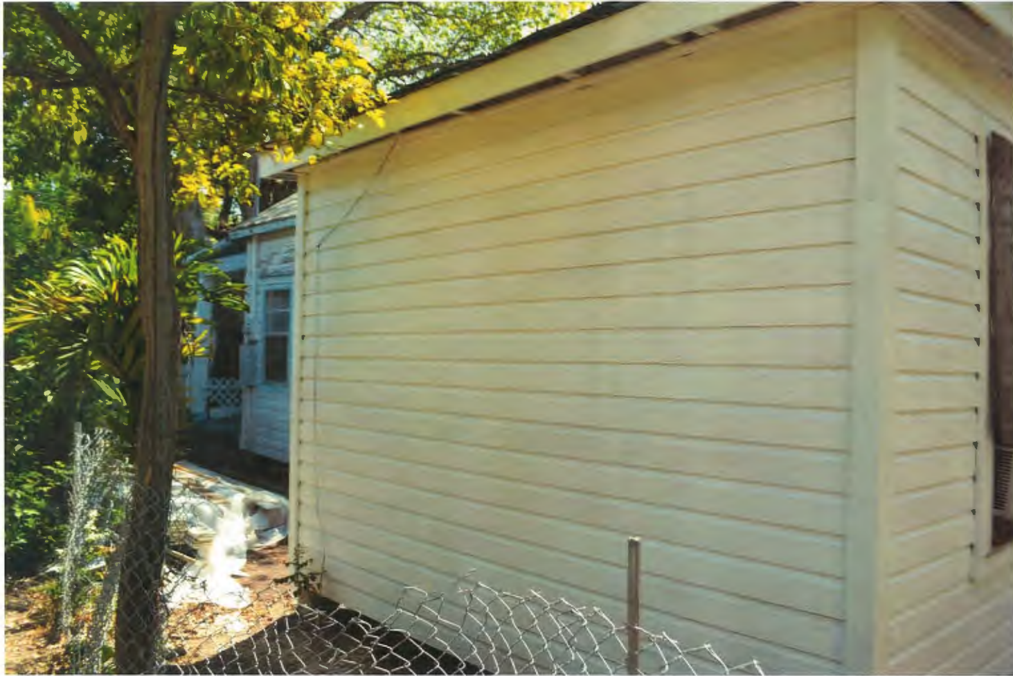
Repaired East Elevation
