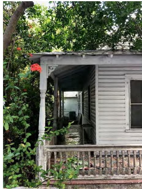
Detail of "L" shape porch.
