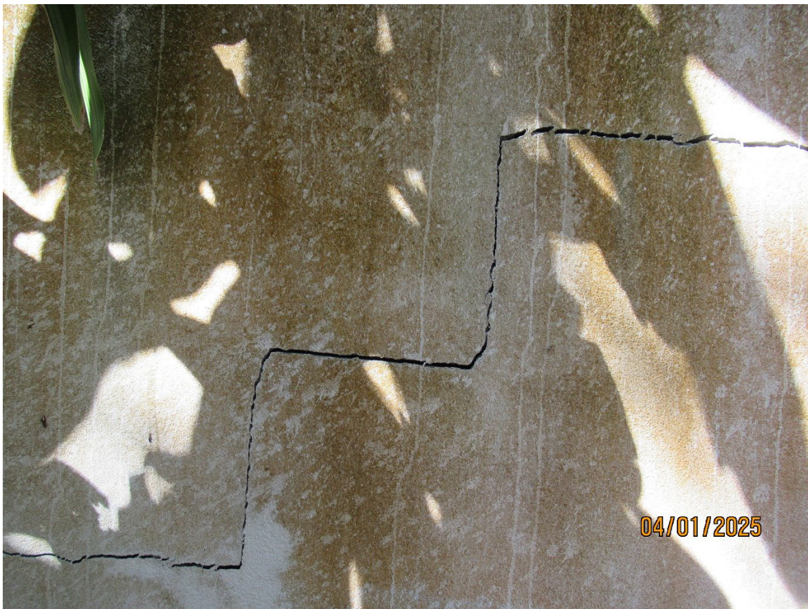
2 photos of the cracking in the concrete wall adjacent to the tree
