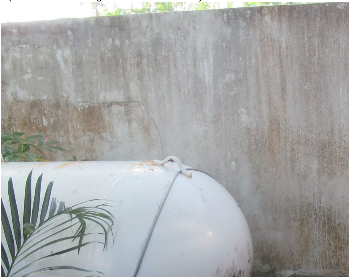
2 photos of the cracking in the concrete wall adjacent to the tree
