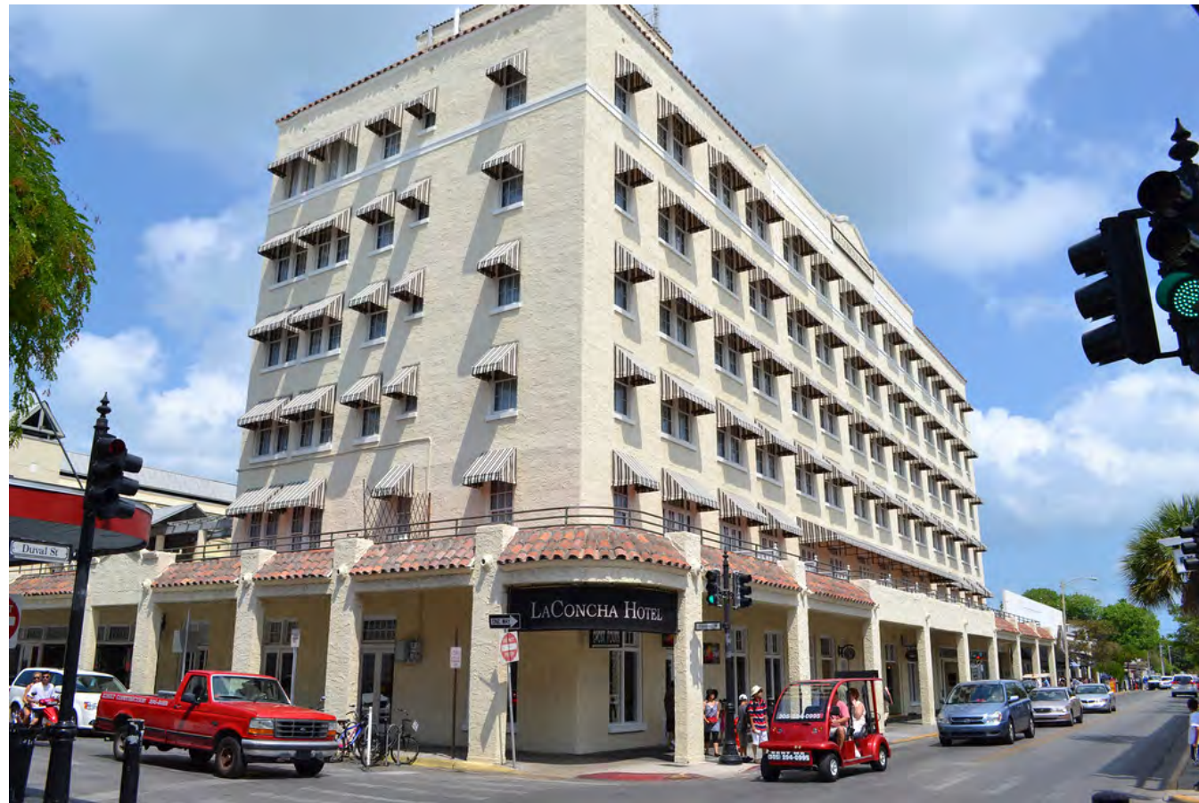
Sign C: Previously installed signage at corner of building. Sign not currently in place.
