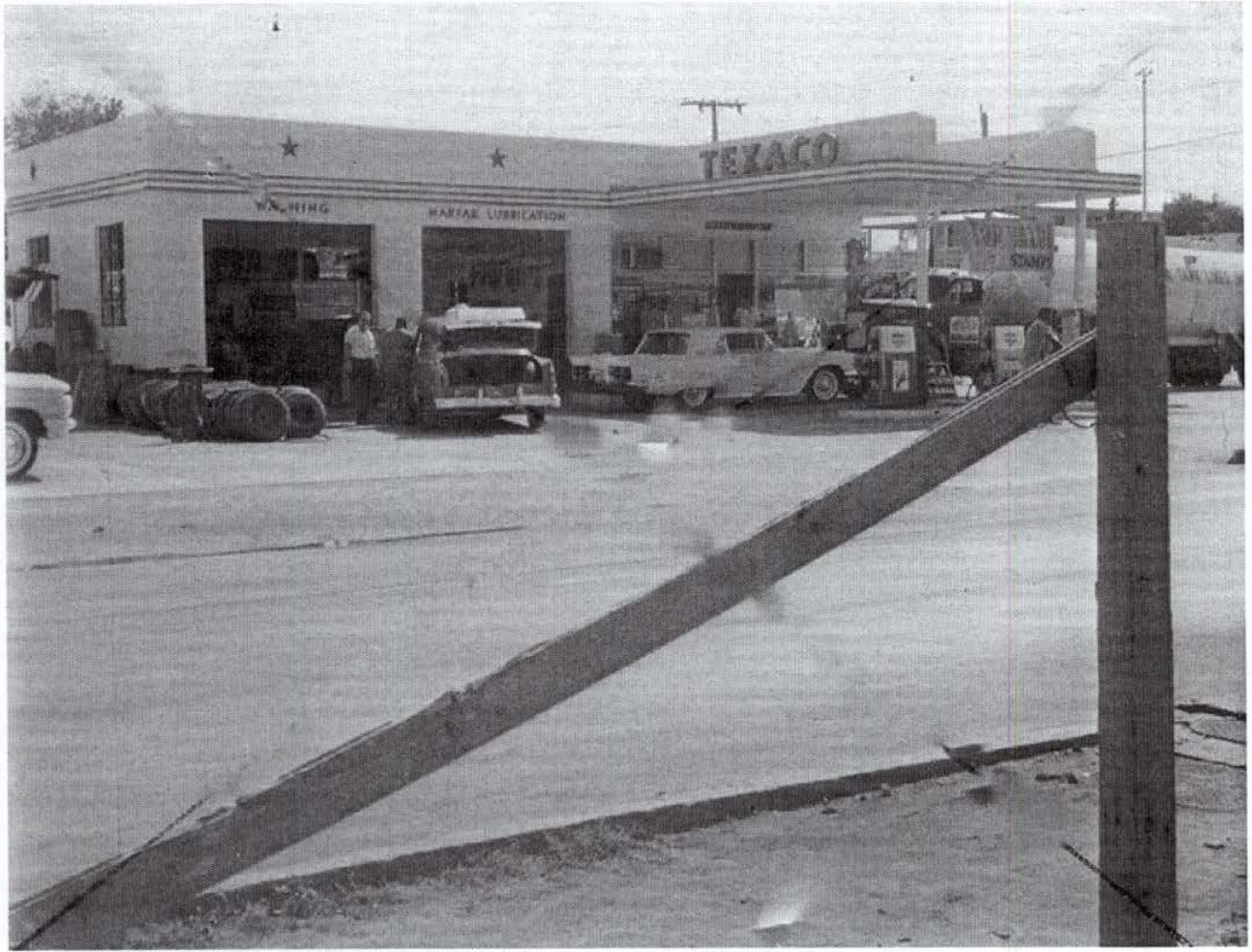
Photo taken by the Property Appraiser's office c1965; 500 Truman Ave.; Southernmost Texaco Service Station; razed about 1972; Monroe County library
