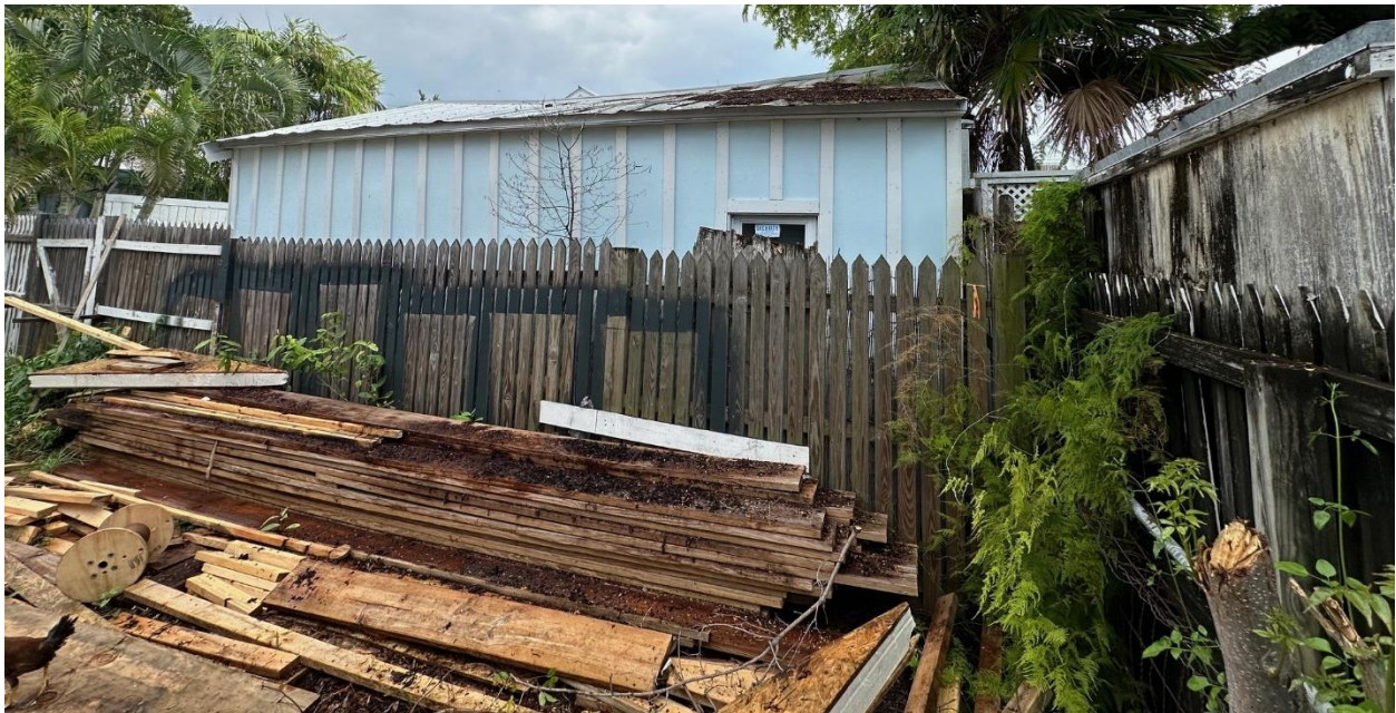
Rear elevation of existing accessory structure. Notice roof's curvature .
