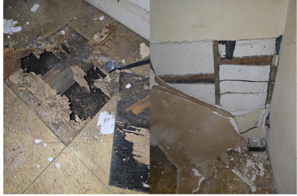
DETERIORATED FLOOR FRAMING & SHEATHING
