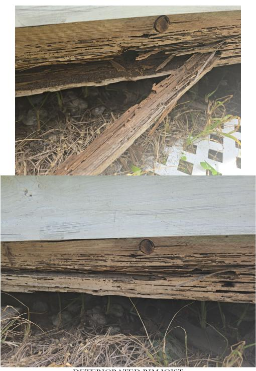
DETERIORATED RIM JOIST
