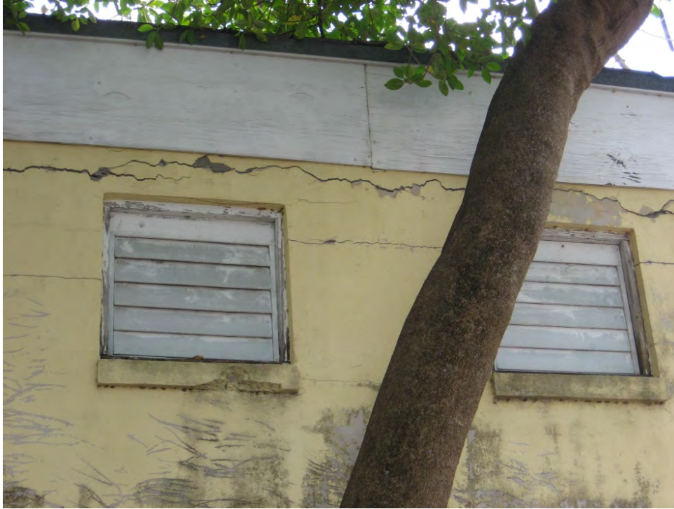
Detail photo of 2 nd floor spalling tie beam at north façade. Contractor to repair spalling at tie beams and columns and patch stucco. See structural details and specifications.
