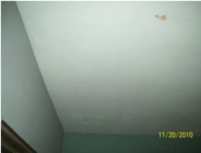
Photos by M. Gonzalez Nov. 20, 2010 Unfinished roof is leaking into neighbor's unit.
