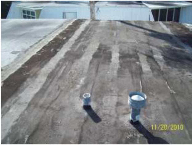
Photos by M. Gonzalez Nov. 20, 2010 Unfinished roof is leaking into neighbor's unit.
