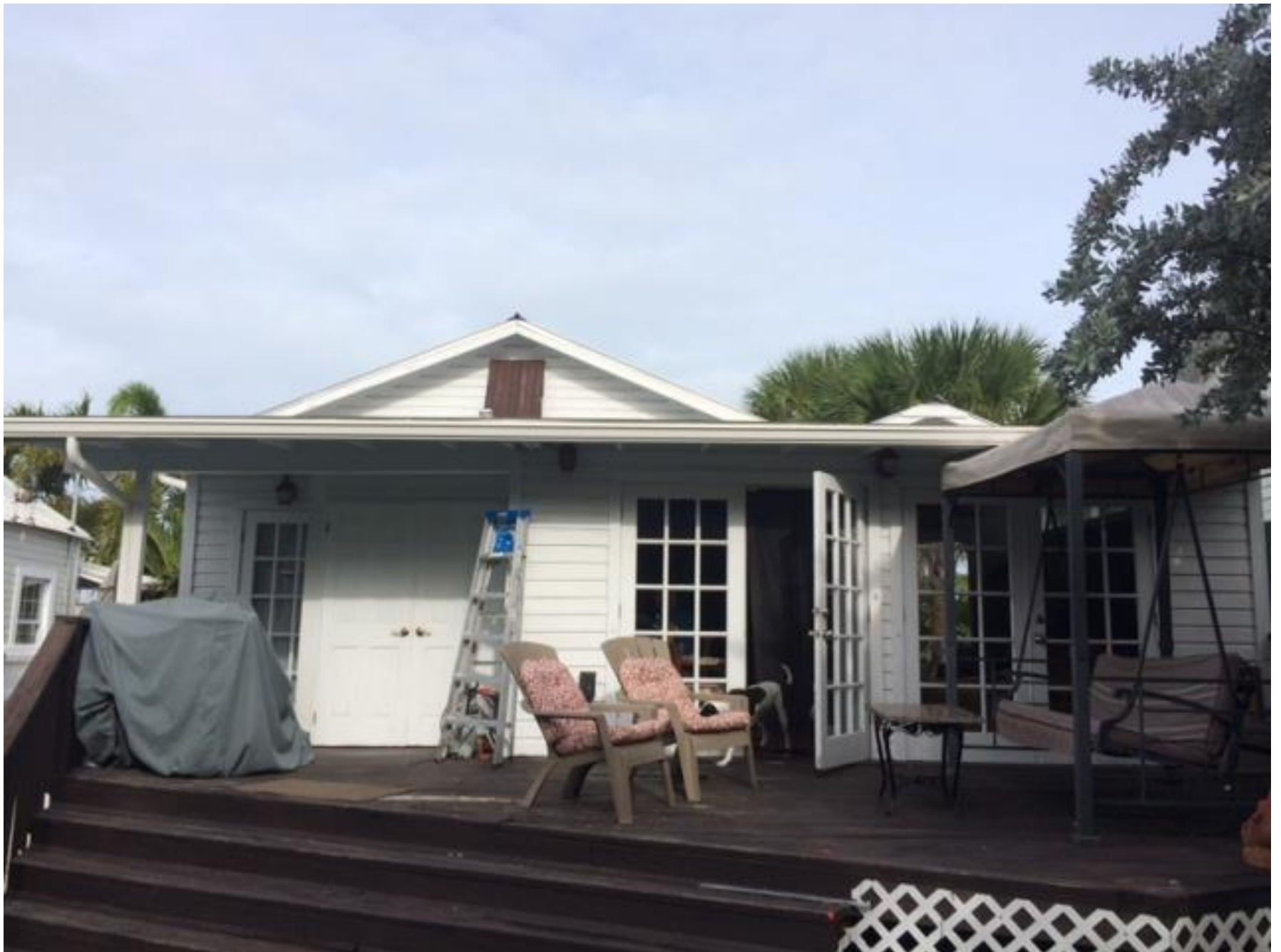
Rear of house
