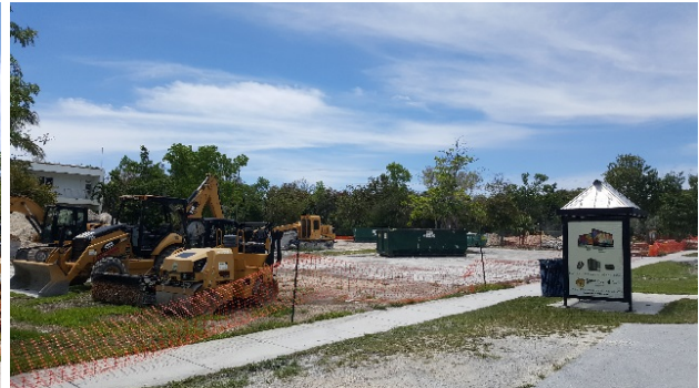
Photograph of the property being cleared
