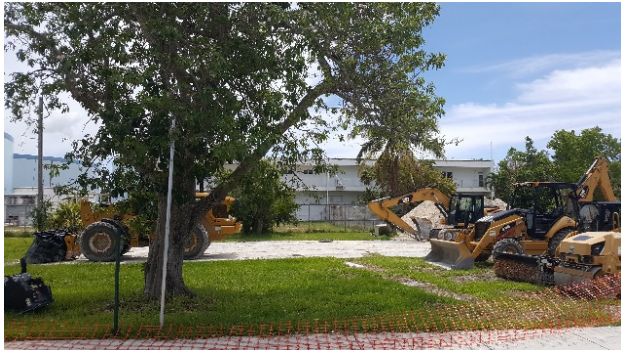
Photograph of the property being cleared
