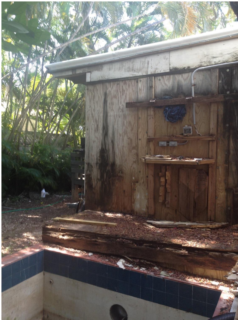
Rear of 818 Sawyers Lane
