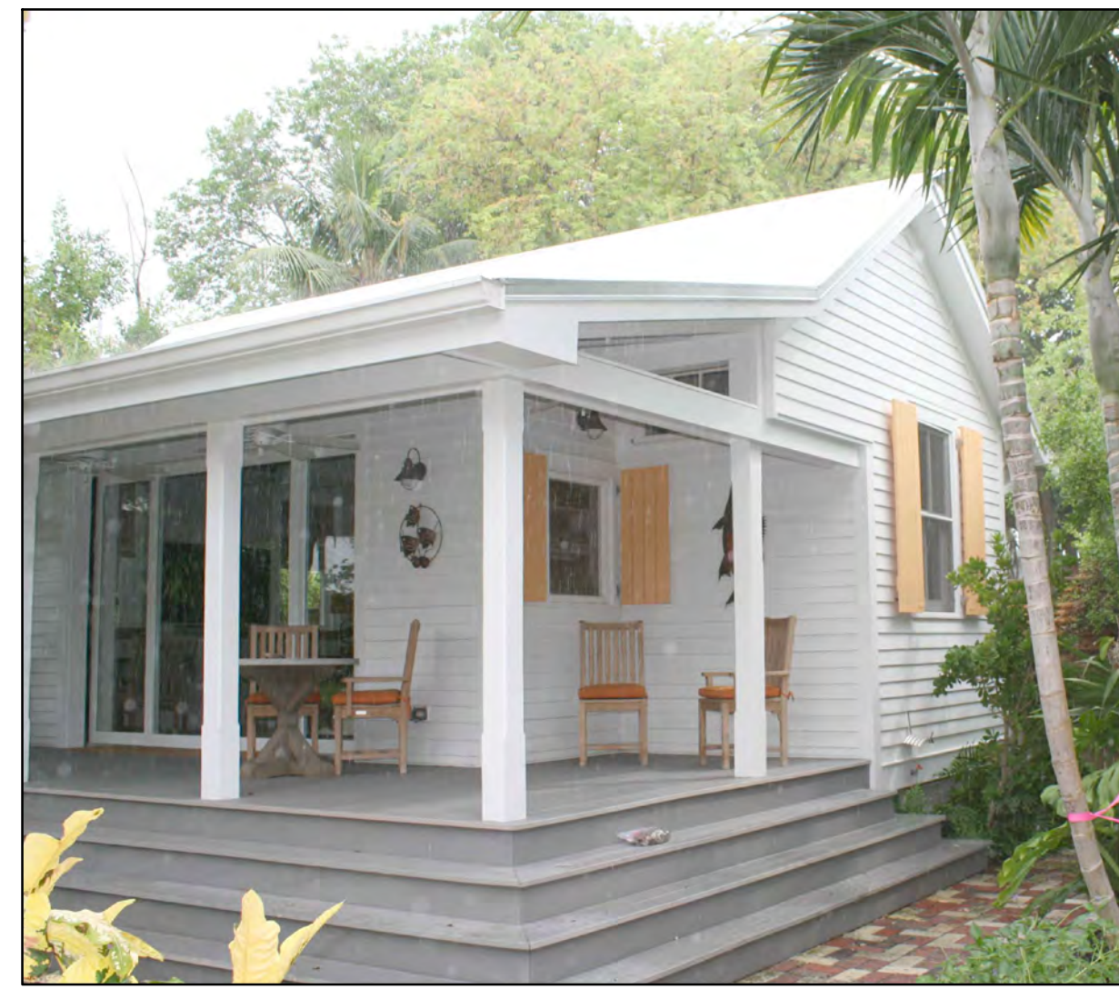
7 PHOTO DETAIL 3 (EXISTING POOL HOUSE) A2.5
