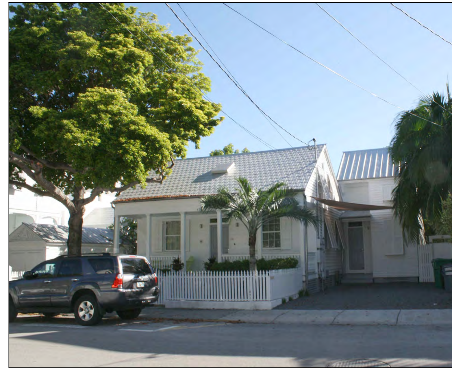
3 PHOTO DETAIL 3 (420 ELIZABETH STREET) A8.0
