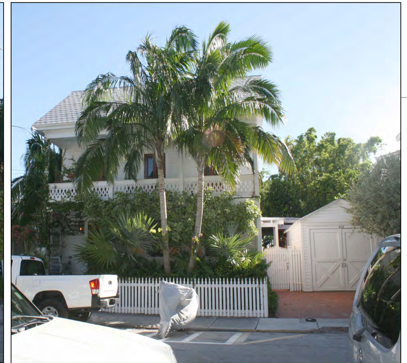
4 PHOTO DETAIL 4 (416 ELIZABETH STREET) A8.0
