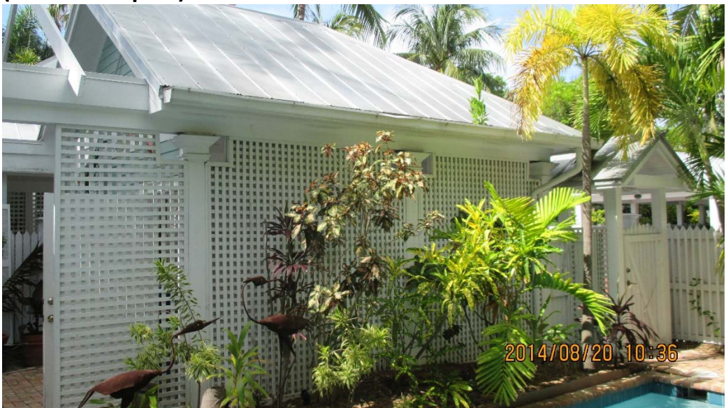
(View of carport)
