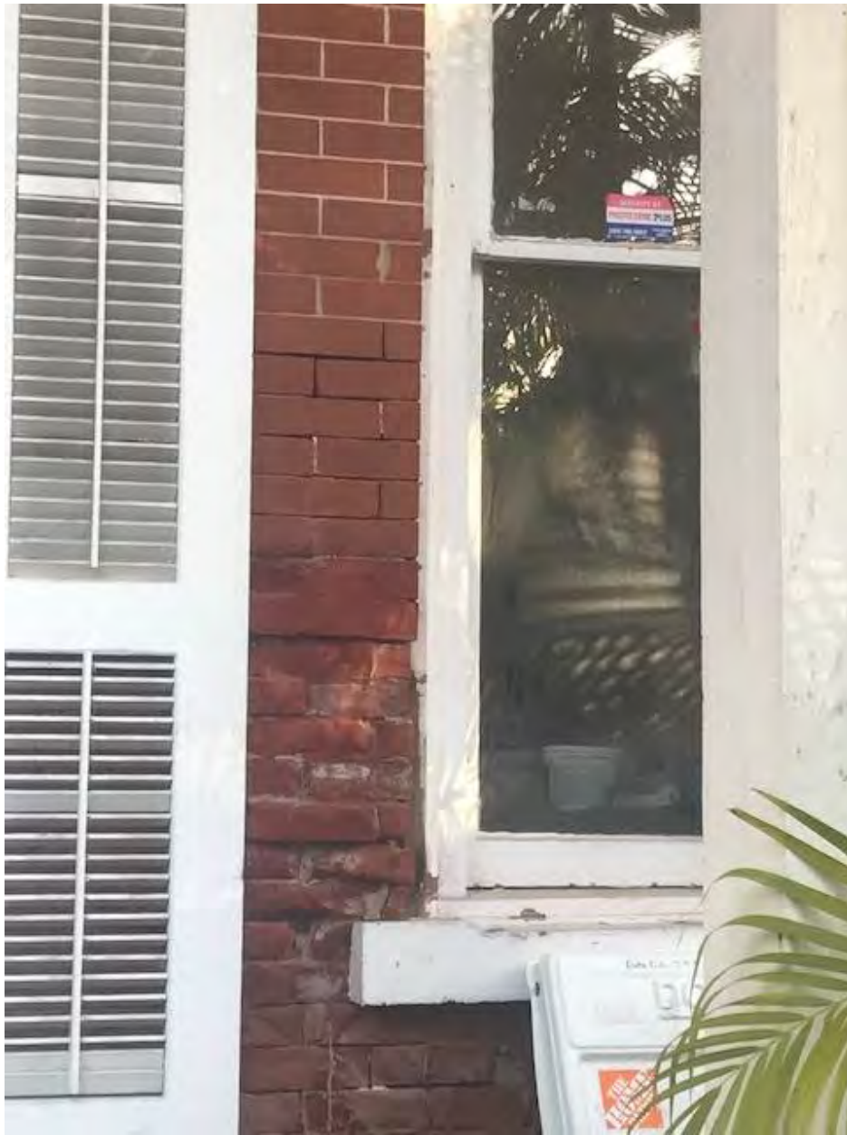
Current conditions, detail front wall.
