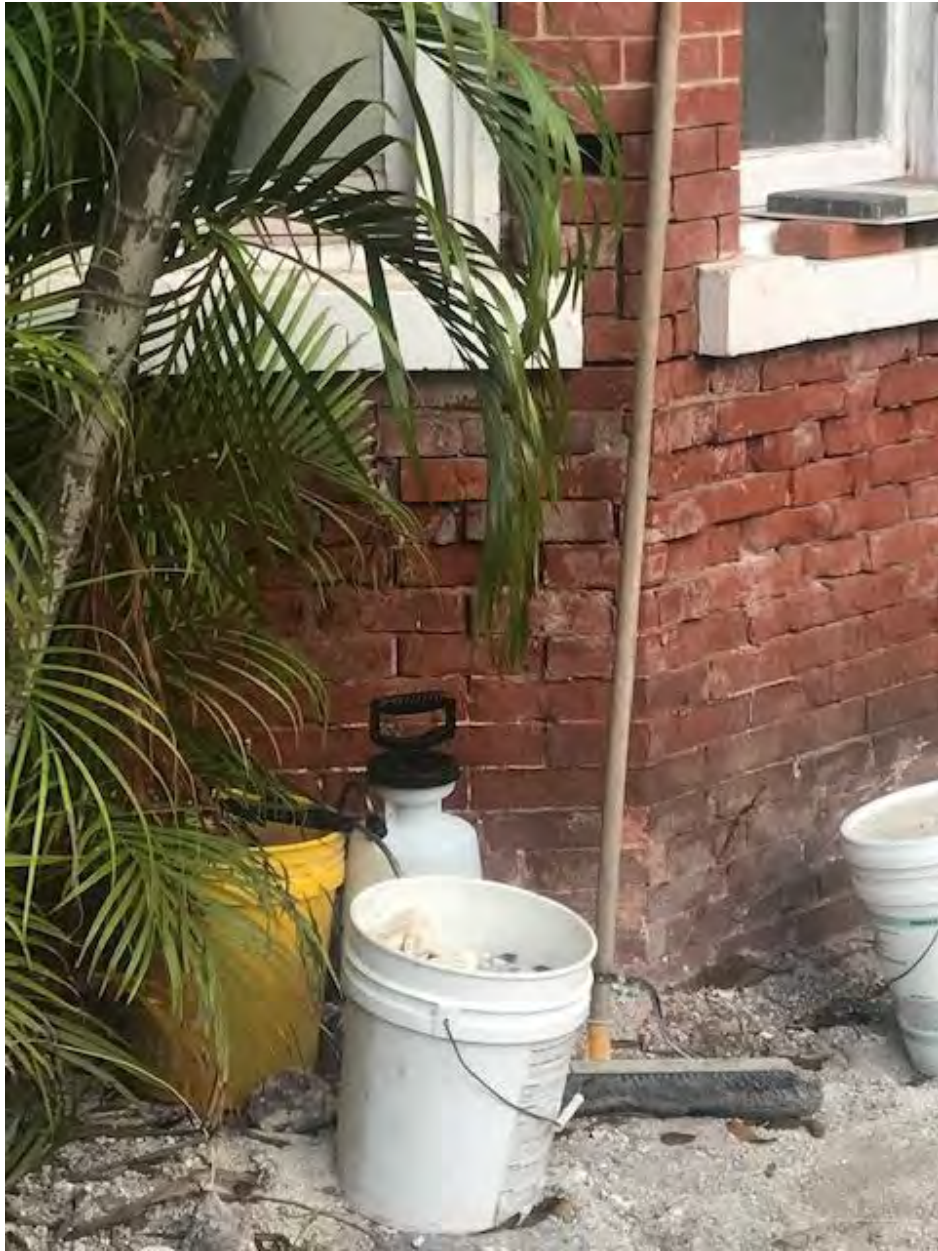
Current conditions, detail of lower portion of turret.
