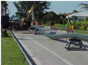
10-inch HDPE FM being pulled through drilled hole.
