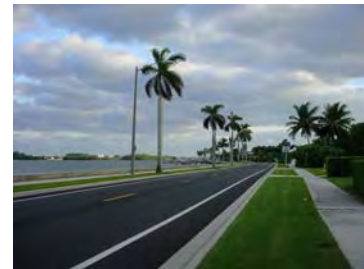
South Flagler Drive after completion of project. The entire road in our project area was micro-surfaced.
