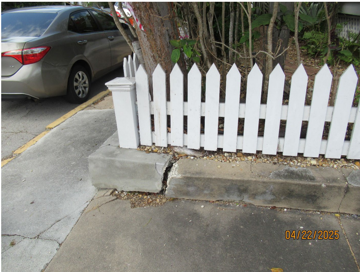
A photo of the wall cracking near the tree and a photo of the wall cracking elsewhere
