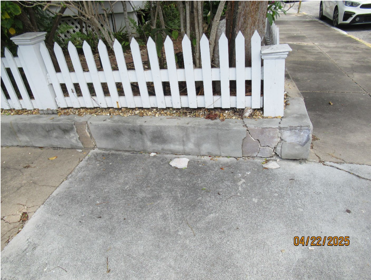
A photo of the canopy of the tree and a photo of the wall cracking near the base of the tree
