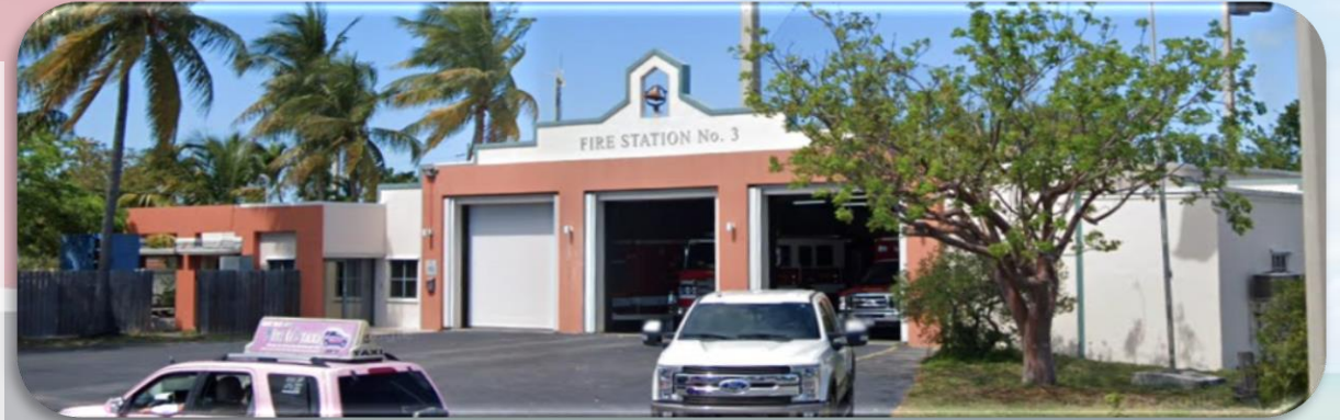
EXISTING FIRE STATION 3
