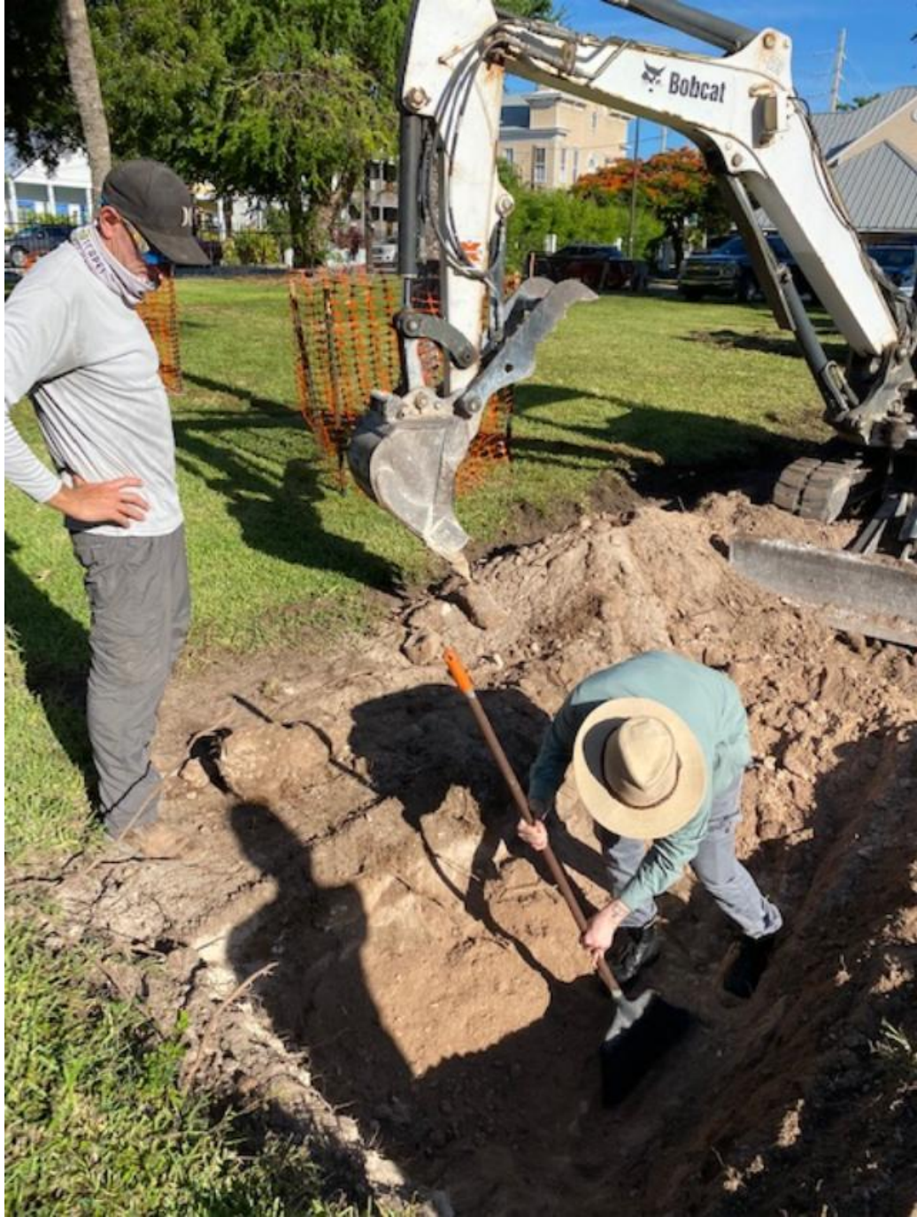
Evan Bell and Malachi Fenn excavating Trench 1.
