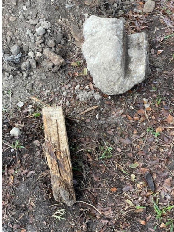
Post fragment in concrete
