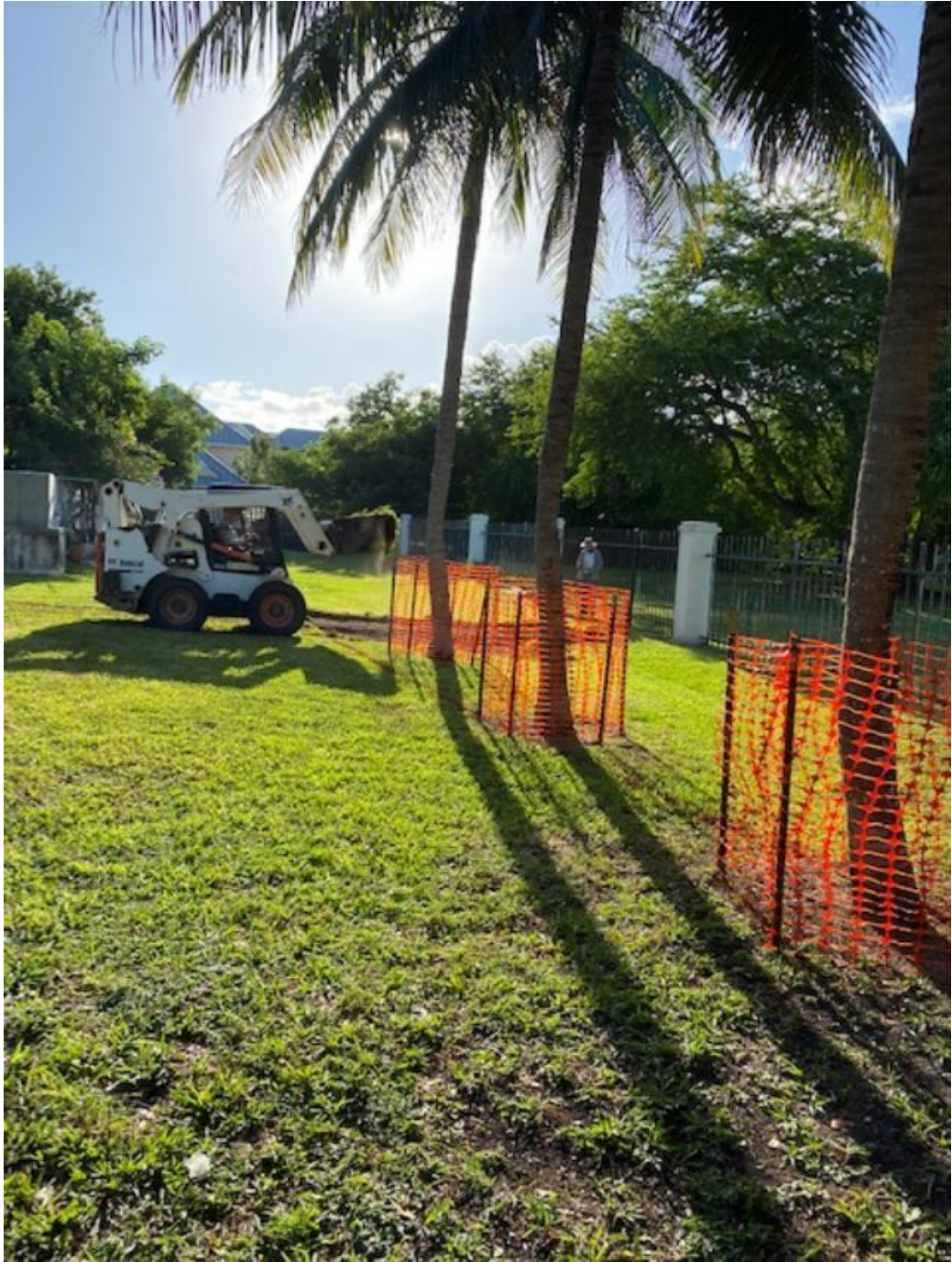
Bobcat used in excavation.
