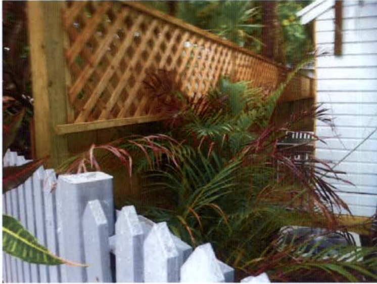
FRONT LEFT CORNER OF HOUSE RED TAGGED FENCE
