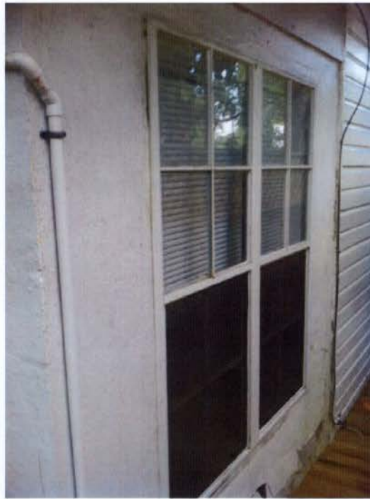
SOUTH WEST SIDE OF HOUSE EXISTING WINDOWS
