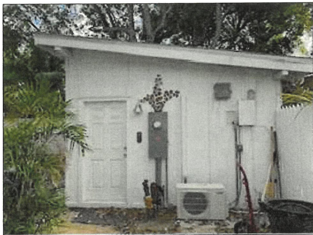
2 VIEW FROM INSIDE OF PROPERTY (EXISTING WEST ELEVATION) A7 SCALE: N.T.S.
